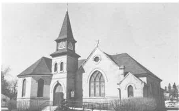
179) Knox Presbyterian Church Construction Date: 1904 Location: Eveline Street, Selkirk Present Owner: Presbyterian Church of Canada Present Use: Active Congregation Construction: walls - buff brick on wood frame roof - asphalt shingles on milled wooden rafters Integrity: Largely unaltered Condition: Good Notes: This building is also discussed on pages 115 and 117.
