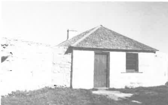
251) Northwest Bastion Construction Date: 1840s Location: Lower Fort Garry National Historic Park Present Owner: Parks Canada Present Use: Display Construction: walls - dressed limestone roof - wood shingles on hewn timber rafters Integrity: The structure has been carefully restored. Condition: Good
