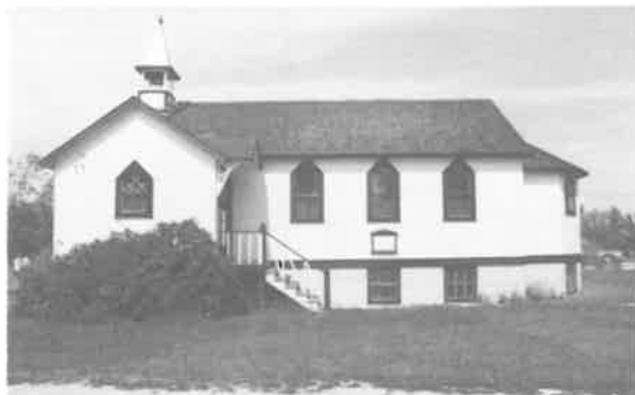
177) St. Peter's-Dynevor Church Construction Date: ca. 1925 Location: River Lot #34 Present Owner: Anglican Church of Canada Present Use: Active Congregation Construction: walls - horizontal siding on milled wooden frame roof - asphalt shingles on milled wooden rafters Integrity: Largely unaltered Condition: Good
