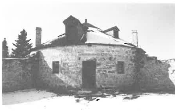
250) Southwest Bastion Construction Date: 1840s Location: Lower Fort Garry National Historic Park Present Owner: Parks Canada Present Use: Display Construction: walls - dressed limestone roof - wood shingles on hewn timber rafters Integrity: The structure has been carefully restored. Condition: Good
