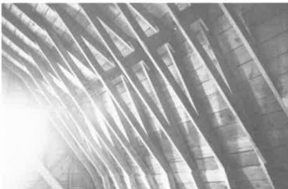
Plate 88. Detail of typical rafter construction in a gambrel-roofed barn.
