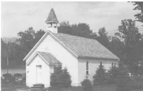
178) St. George's Anglican Church Construction Date: 1938 Location: St. John's Boy's School/River Lot #41 Present Owner: St. John's Cathedral Boy's School Present Use: School Use Construction: walls - horizontal siding on milled wooden frame roof - asphalt shingles on milled wooden rafters Integrity: The church has been moved onto its present site. Condition: Good
