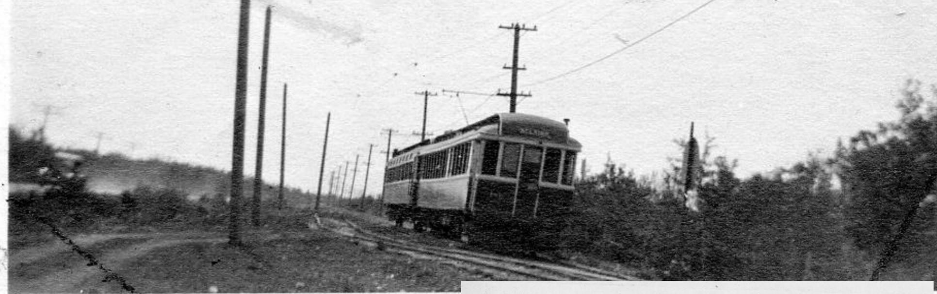
Road bed was quite rough as it was laid on a minimal road bed with little ballast and the cars rocked violently as they sped down the tracks at 30 miles per hour.
