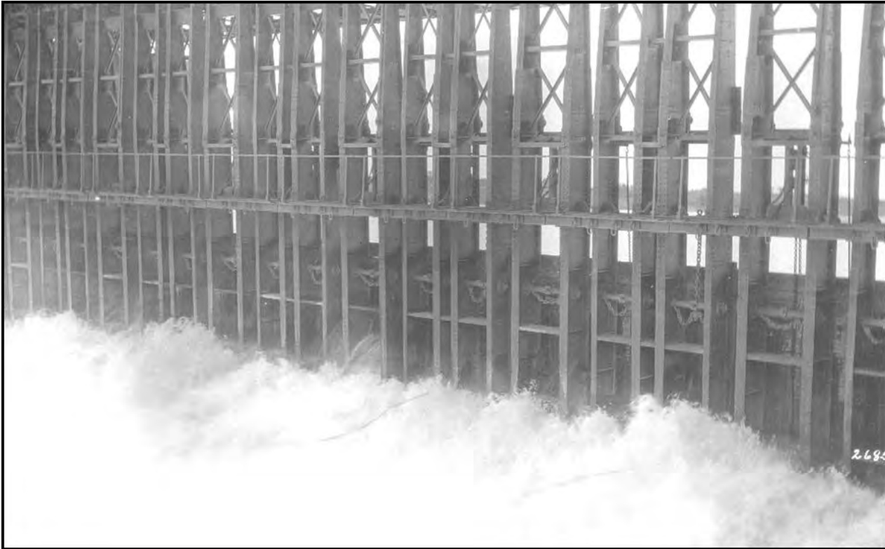
Steel frames weighing approximately 10 tons, are lowered into the water and the moveable wood lath gates are lowered into the frames to hold the water back.
