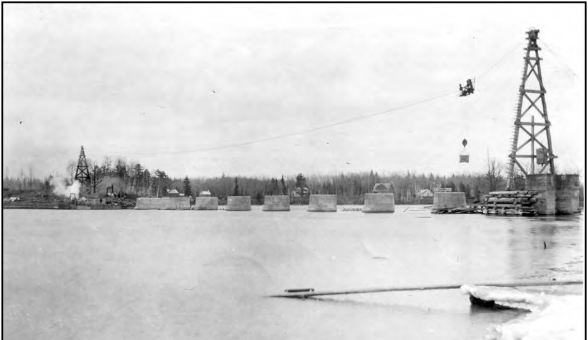
Cable tram ways were used to move concrete and other materials across the dam during construction
