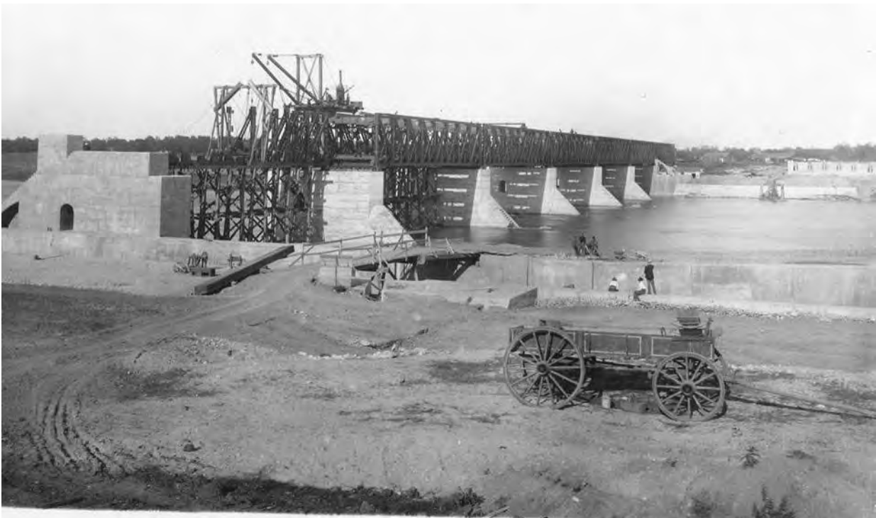
Steel frames being constructed that would contain the wooden roll curtains that formed the actual movable dam. Each curtain is made up of 50 Douglas Fir laths fitted into a heavy cast iron plate at the bottom. The frames weigh between 5-9 tons and are dropped to the concrete frame at the bottom of the dam. They can be adjusted according to river flows.
