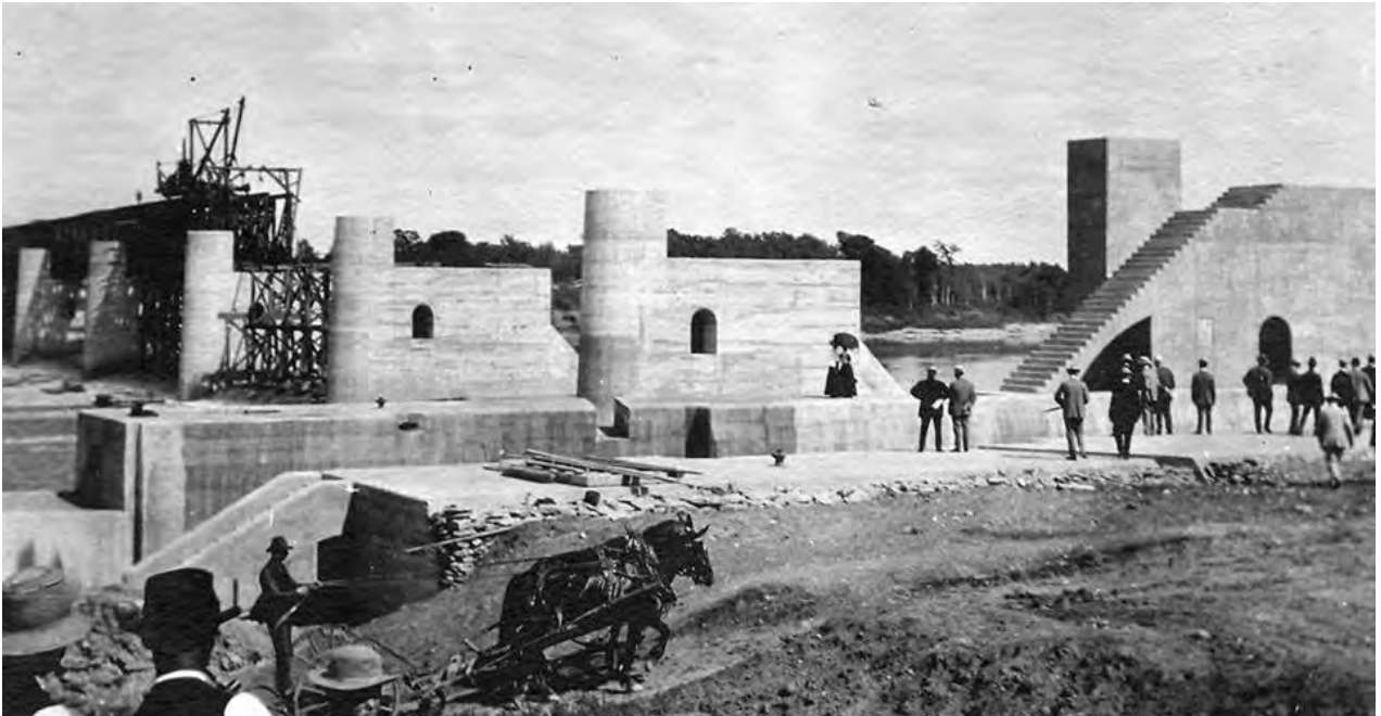
The seven bridge spans were erected in the summer of 1909 each with trusses 21ft wide x 126ft long.
