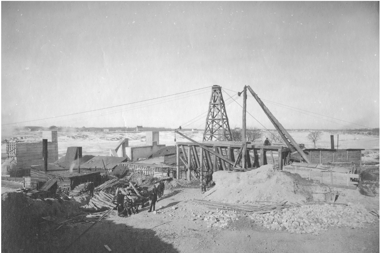
Most of the excavation work was accomplished in the winter months – provided the frost was not too severe
