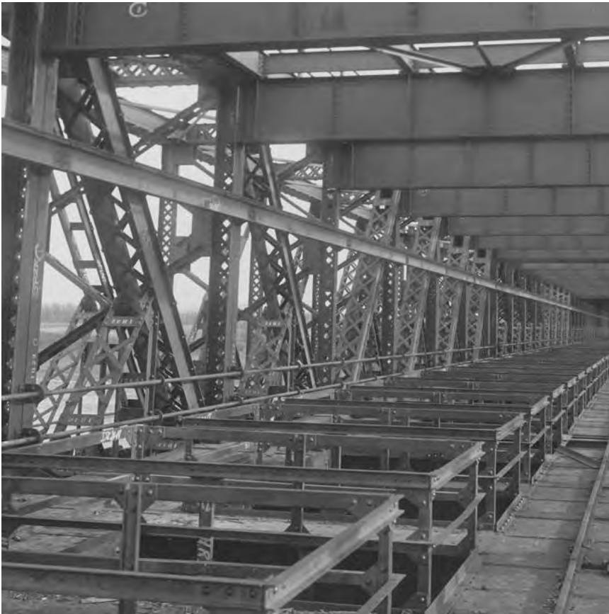
Large open bays provide access for attaching and removing the curtains each of which are made up of 50 Douglas fir wood laths 7 ft wide and 13ft long which can be rolled up or down depending on the required water height.
