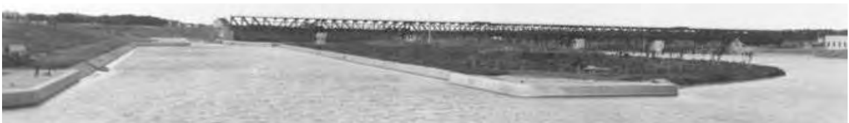
Views of the upstream approach to the lock, taken from the bridge and from on board an excursion steamer. The concrete abutment at centre acted as an ice breaker during the spring melt to help minimize damage to the structure as the ice flows passed through the open dam gates. Although the old time steamers are long gone, boating excursions are still popular. The Island was created from mud from the base of the dam.
