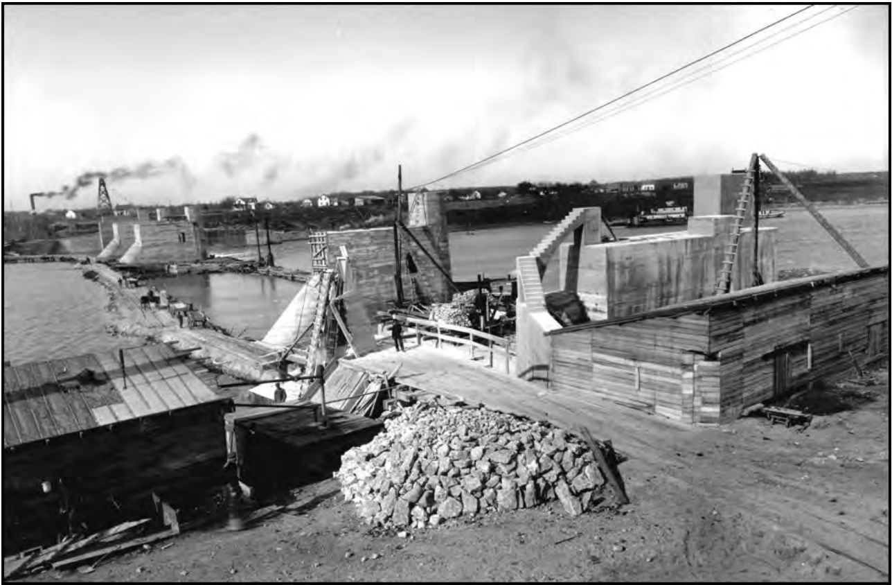
View of the main piers under construction. Note the temporary causeway / roadway located on either side of the row of piers and the tower and the cable mechanism used to carry huge buckets of concrete from the shoreline to the piers. (Manitoba Archives Photo.)
