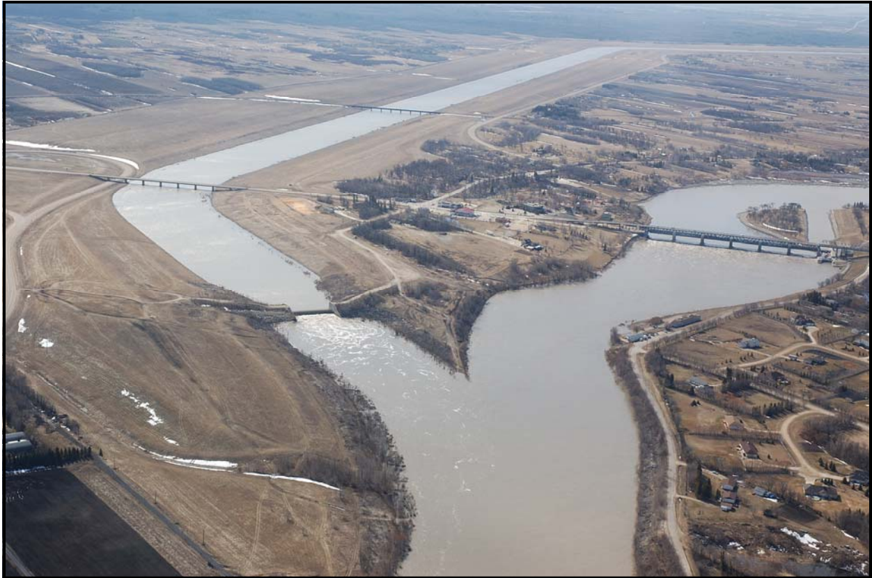
View of the Red River Floodway outlet located just downstream from the Lockport Bridge and Dam. In this photo, the floodway has been opened during the spring melt. Normally the floodway channel would contain a trickle of water, particularly during the summer and autumn when river water levels are naturally low.
