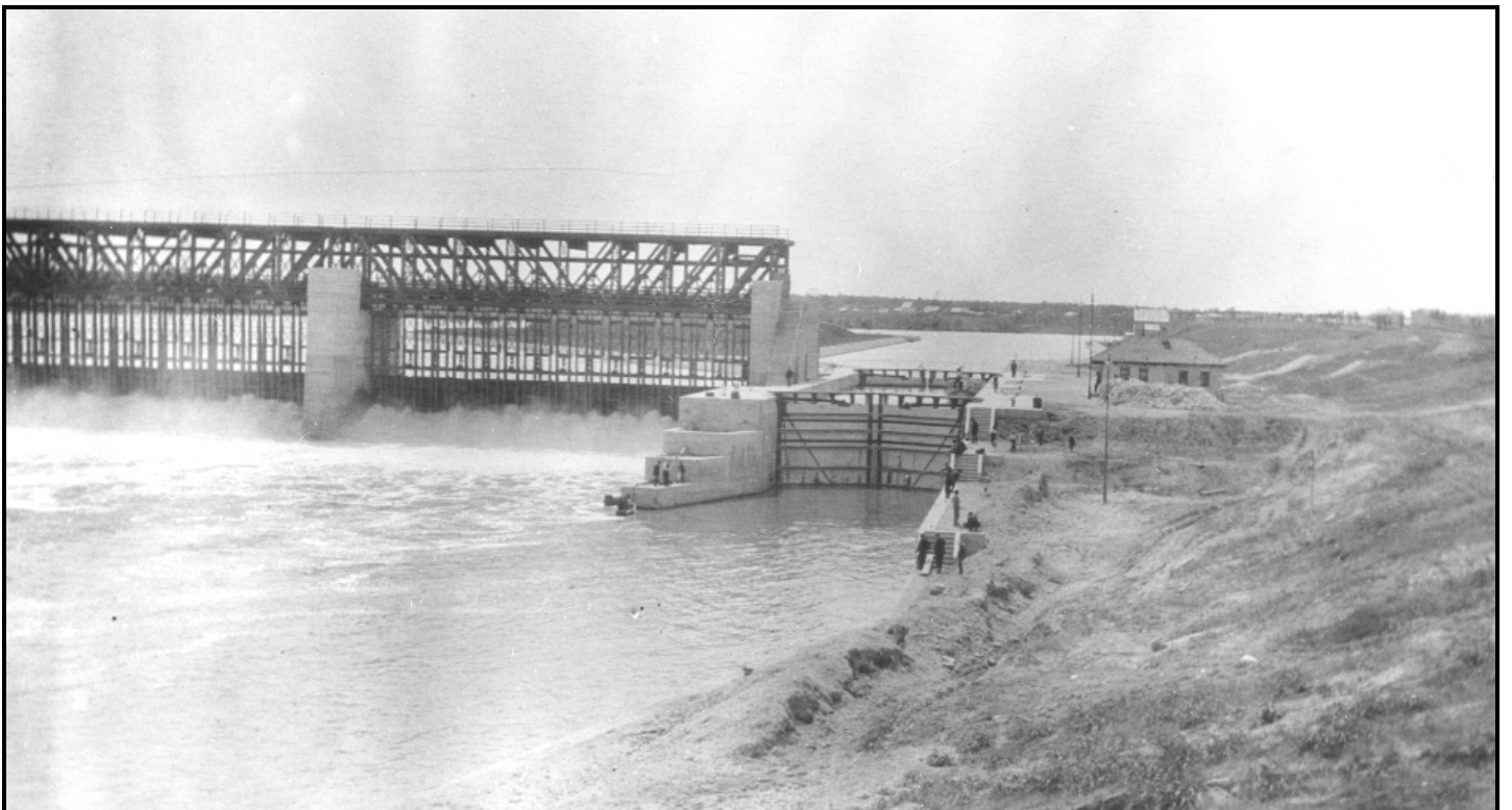
Above and below: Two excellent views of the lock and dam soon after its completion in 1910. The roadway decking and approaches have yet to be constructed at the time of these pictures. Note the people fishing on the downstream side. (Manitoba Archives Photo.)
