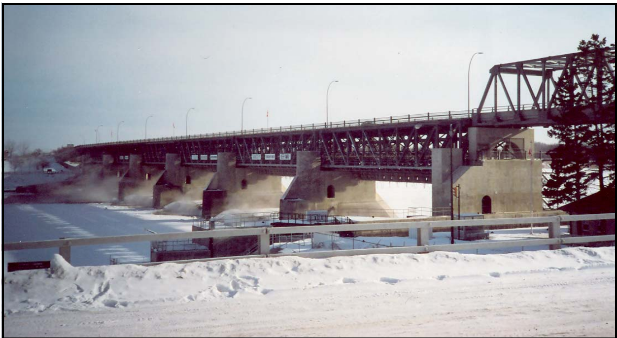
Views of the dam and bridge during the winter. Note that the curtains are in their fully retracted position.
