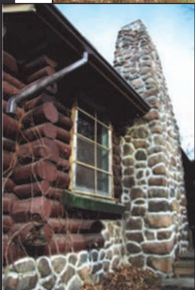
Saddle Notch Construction Detail
