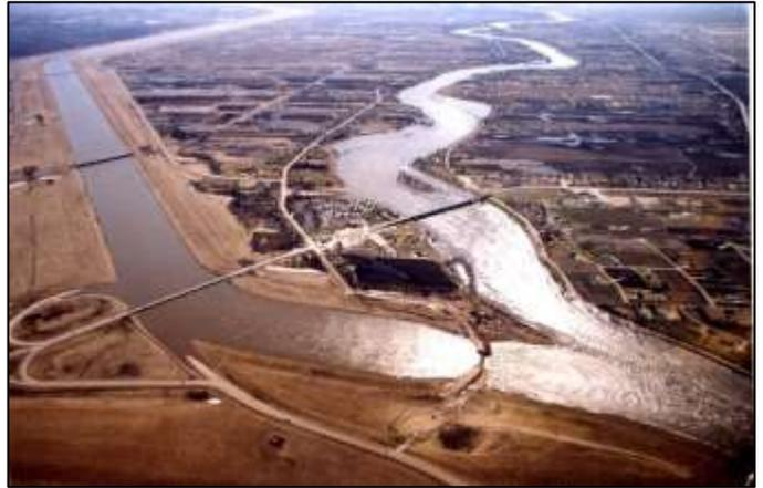
It can divert up to half of the Red River's spring flood water around the City of Winnipeg running just south of St. Norbert and during flood periods, takes part of the Red River flow water around Winnipeg to the east and discharges it back into the Red River below the dam at Lockport; 47kms (29 miles) long.
