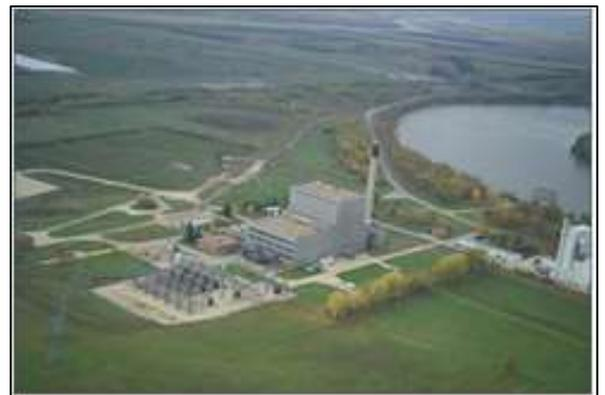
The location was chosen for availability of adequate water supply from the Red River: 144,000 gallons of water per hour are pumped in for cooling and then discharged into Cooks Creek. The 2 wells drilled on the site are over 73 m or 240 feet deep and supply the necessary water for domestic and bearing cooling purposes as well for the boilers.
