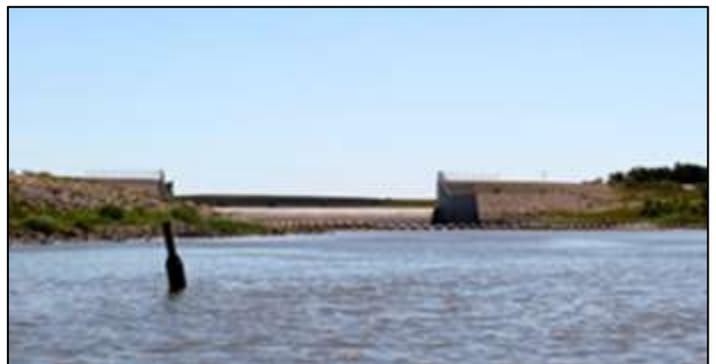
Over time portions of the floodway were compromised so in 2014, a \$627 million floodway expansion program was completed which involved rebuilding the outlet at Lockport; improvements to the Inlet Control structure, raising train and highway crossings and increasing the floodway capacity to allow a flow rate of 4,000 cubic metres (140,000 cubic feet) per second, the estimated level of **a one-in-700 year flood event.**
