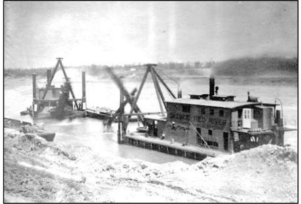
In more recent years, dredges involved a more modern suction system where a snorkel like tube with cutting bits on the end would dig into the river bottom and then with water, pump the sediment through a long pipe to the edge of the river bank.
