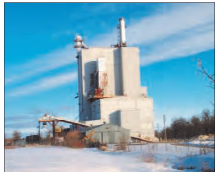
Dow Corning plant
