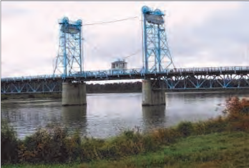
Selkirk Lift Bridge
