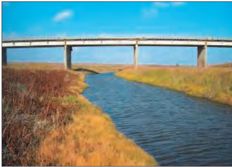
Red River Floodway, Lockport
