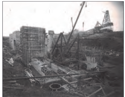
Lock and Dam construction
