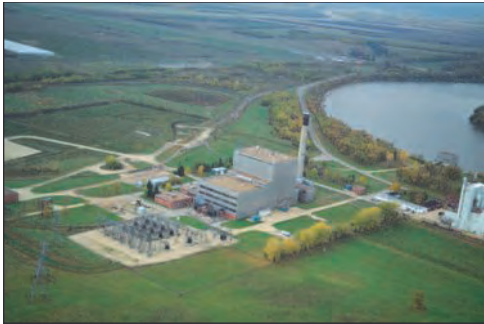
Selkirk Generating Station
