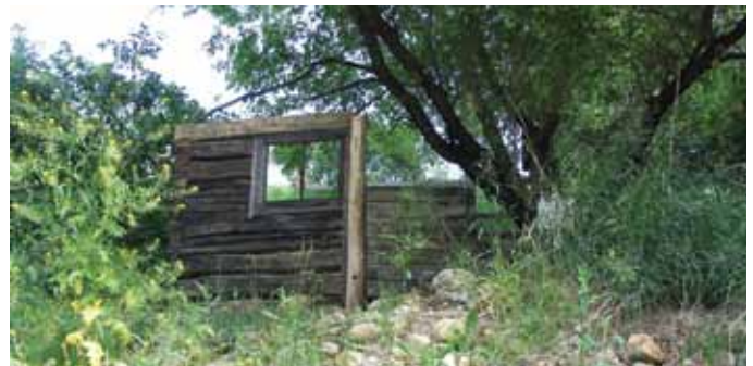
The character-defining elements of Doukhobor Dugout House NHSC in Saskatchewan, such as the window frames, had suffered visible deterioration from exposure to the elements. A long-term repair solution was necessary to prevent further decay and to preserve the site's heritage value.
