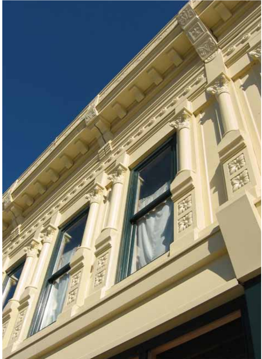
Detail of pressed metal facade after rehabilitation, showing the hallmarks of the original Mesker design. The work consisted of the following: removal of the metal panels, carefully identifying their original locations; removal of multiple layers of paint using a chemical bath; recoating with an epoxy-based paint system; and reinstallation in the original locations on furring strips according to a rain screen principle.
