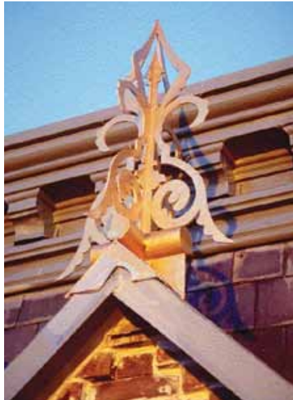
Under certain circumstances, substitute materials may be appropriate. As part of a Rehabilitation project, new finials were designed based on original remains. The originals were fabricated of wafer-thin galvanized metal soldered together. The substitute material used in the new design was plate aluminum.
