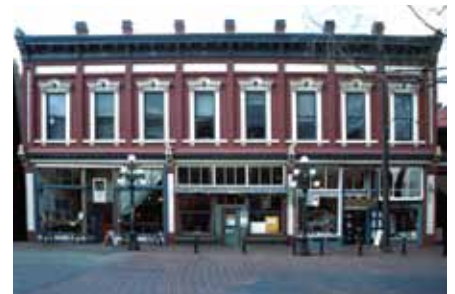
The character-defining form and features of the Byrnes Block storefronts in Gastown, Vancouver, including their large plate-glass display windows with multi-pane transom windows above and recessed central doorways, have been retained through Preservation.
