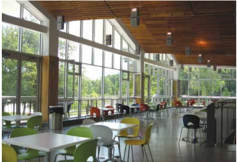
Wood was often used in modern buildings as a finish to contrast with more industrial materials, or as part of an acoustical treatment on ceilings and walls. The wood ceiling and column claddings of the Beaver Lake Pavilion in Montreal were carefully preserved as part of the recent rehabilitation of the pavilion.
