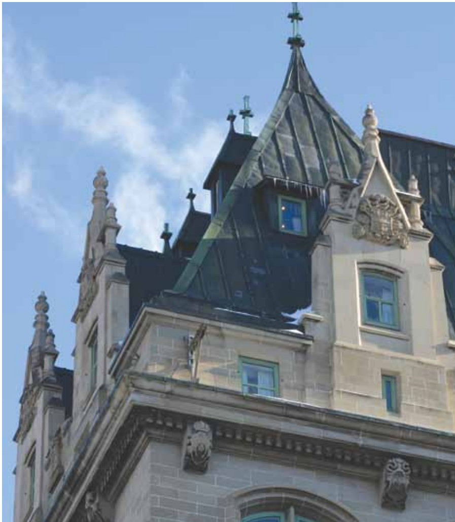
The steep copper roof of the Fort Garry Hotel in Winnipeg is defined by a multitude of small shed- and hip-roofed dormers, highly elaborate stone dormer facades at the corners, a wealth of pinnacles and large ornate chimneys.
