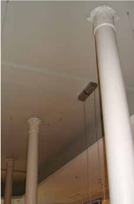
These cast iron columns were uncovered and restored when CentreBeam Place, in St. John, was rehabilitated.
