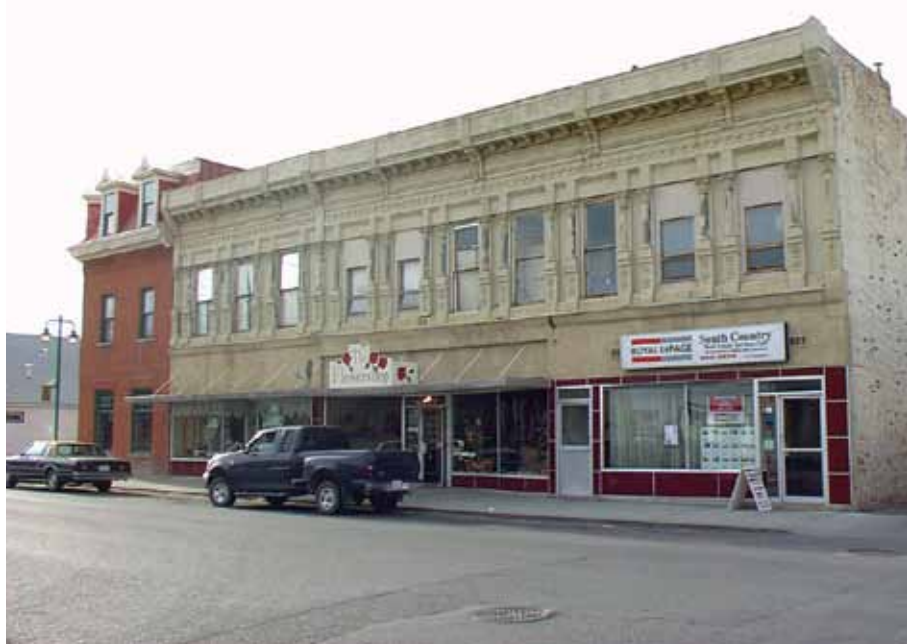
Before rehabilitation: east façade, looking southwest.
