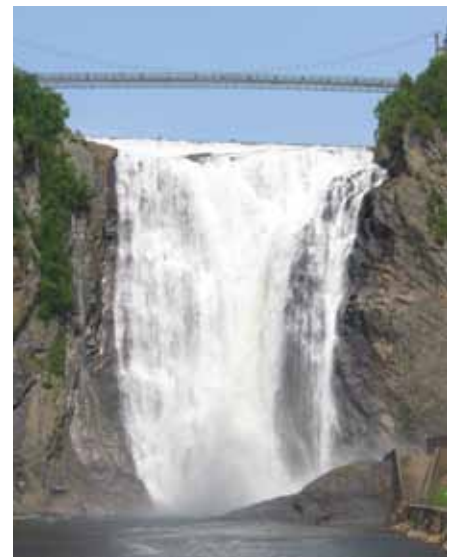
The bridge over the falls.
