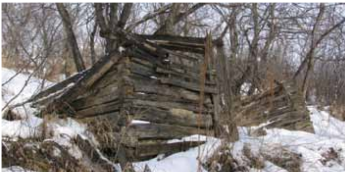
The character-defining elements of Doukhobor Dugout House NHSC in Saskatchewan, such as the window frames, had suffered visible deterioration from exposure to the elements. A long-term repair solution was necessary to prevent further decay and to preserve the site's heritage value.
