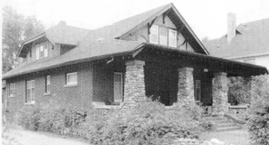
56. 1234 Lorne Avenue, Brandon, 1913. The character of the bungalow comes not from applied style details but from its materials (cobblestone, brick and stucco), structural elements (purlins, piers and brackets) and form (overhanging roof).
