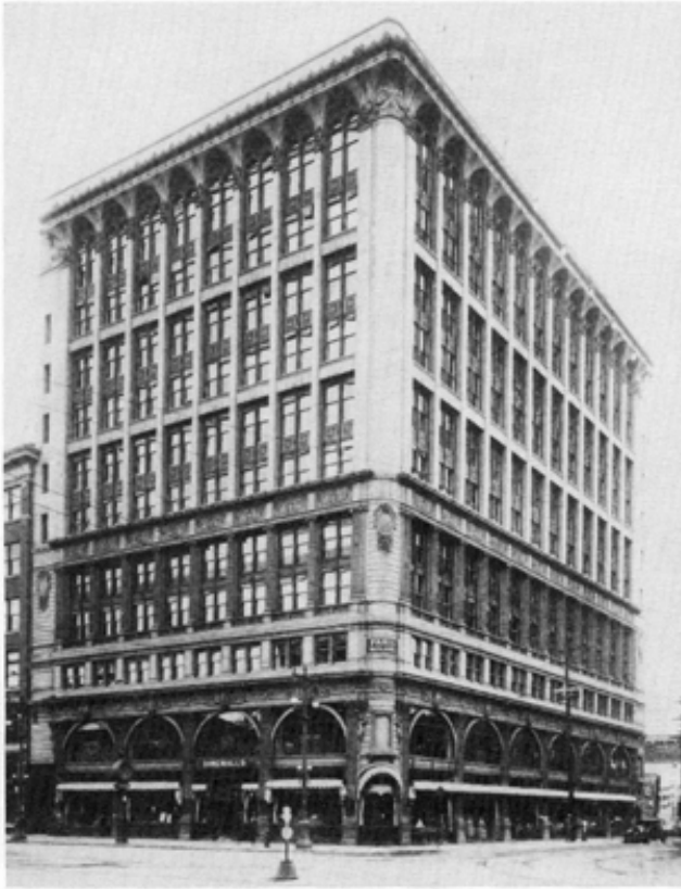
43. Paris Building, Winnipeg, 1915-1917. Because the building was first built as five storeys, there is a stronger horizontal emphasis in the lower floors and a shorter vertical sweep in the piers of the upper floors.
