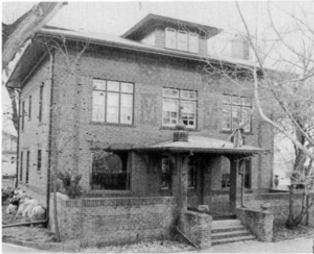
46. Former Post Office, Stonewall, 1914-1915. This use of the Prairie school for a government building is unique in Manitoba. Horizontal emphasis comes from repeated raised bands punctuated by short verticals, rather than a broad eaves overhang.
