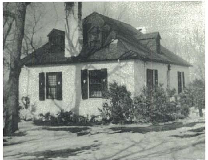
Victoria Cottage in 1982 (east side).
