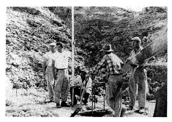
Selkirk Generating Station Project: Levels are checked prior to pouring the concrete, 1957.
