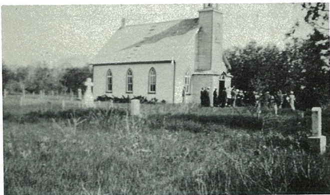
St. James Anglican Church at Poplar Park.
