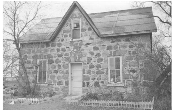
Above: A pioneer home near Brandon constructed using stones collected from the fields (and thus called fieldstone). Below: A detail view of Kennedy House near Lockport (1866) shows the kind of finish required for early stone buildings – thick mortar was used to cover and overlap oddly-shaped stones, ensuring a solid wall.
