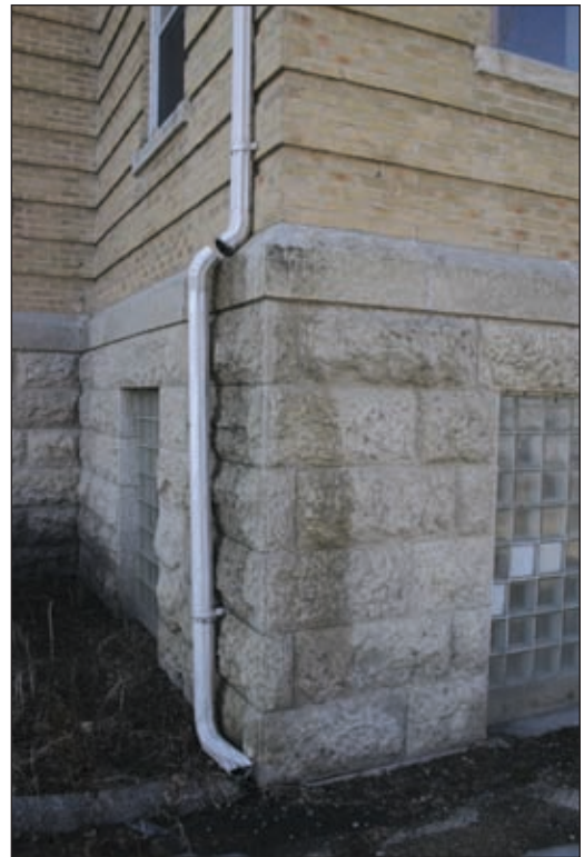
This downspout has come detached between the first and second floors making it completely ineffective. Also it is missing a leader to direct the water away from the building, which would cause foundation damage.
