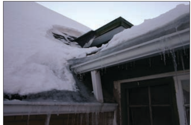
The ice has been allowed to build up at the eaves, potentially damaging the roof line. The best remedy is to improve the insulation in the attic and seal any leaks.
