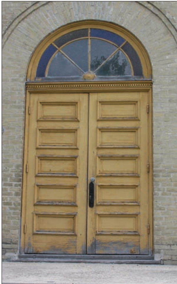
This door needs a new coat of paint to retain the original integrity. The weatherstripping should also be inspected.
