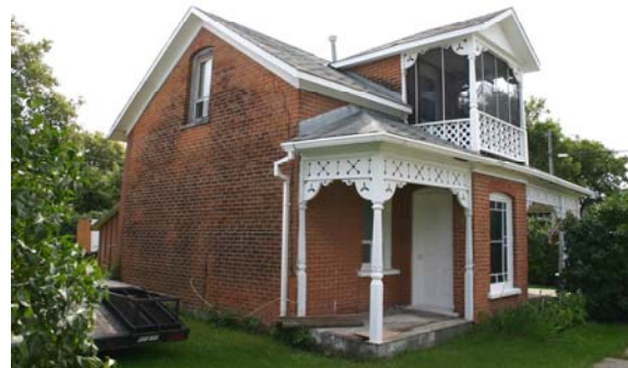
The wealth of details suggests a “Victorian Vernacular.” This example has a protruding central bay and fretwork, but they may vary considerably in plan and elevation, with a range of window types, but typically with some form of gable roof.
