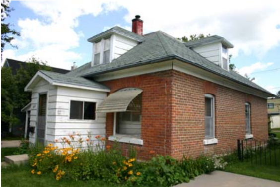
The “Cottage-style” House has a centre-hall plan, dormers and a hipped roof.
