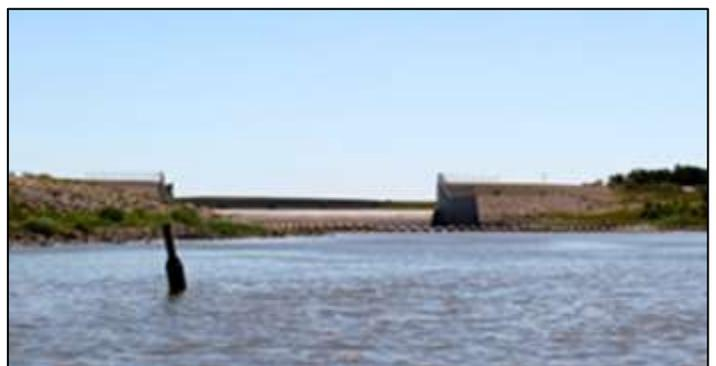
Over time portions of the floodway were compromised so in 2014, a \$627 million floodway expansion program was completed which involved rebuilding the outlet at Lockport; improvements to the Inlet Control structure, raising train and highway crossings and increasing the floodway capacity to allow a flow rate of 4,000 cubic metres (140,000 cubic feet) per second, the estimated level of **a one-in-700 year flood event.**
