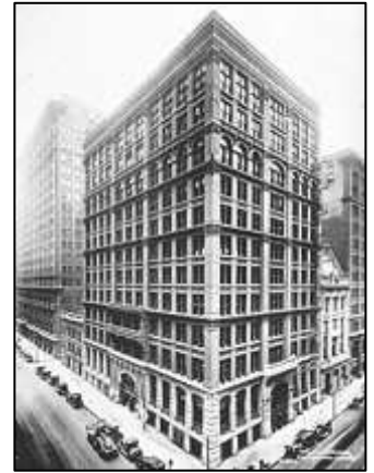
Home Insurance Building, Chicago (1885, demolished) considered the first skyscraper in the world
