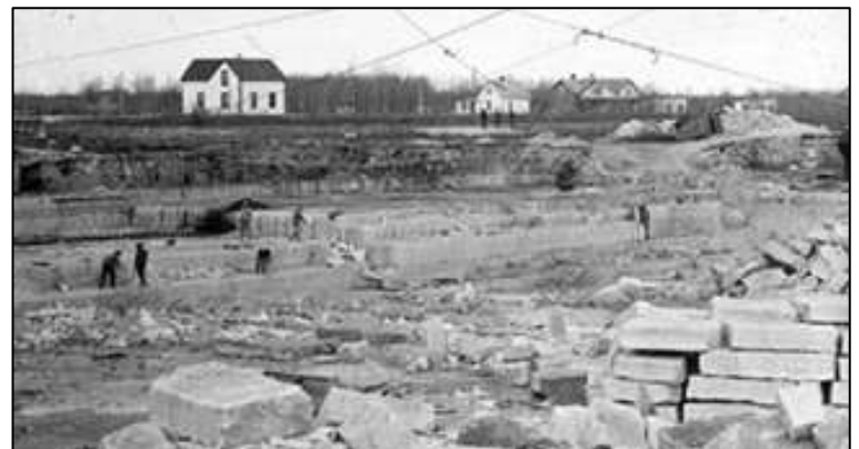
Riverbank Limestone Quarry
