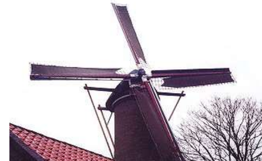
Zierikzee windmill in the Netherlands, showing the placement of sail cloth that allows the mill to attain ongoing productivity even in low winds.
