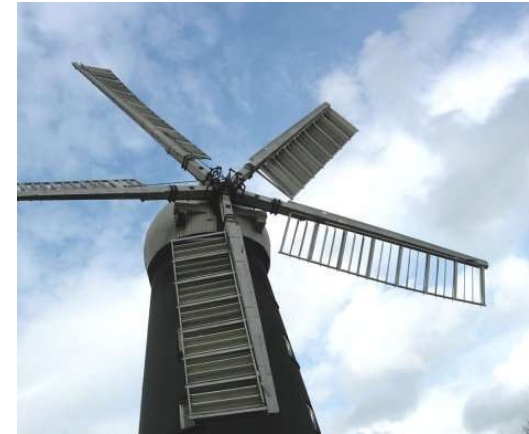
View of the sails on a rare five-sailed tower windmill built in the early nineteenth century.
