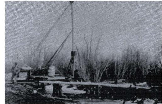
Besides his work as a mechanic (and woodsman and thresher operator), John Bunio built small bridges, as did other entrepreneurial men in the municipality. This image shows the bridge-building technology of the day, used throughout St. Clements to build small culvert-type bridges. Note the pile driver used to sink main vertical supports.
