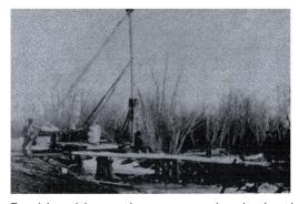
Besides his work as a mechanic (and woodsman and thresher operator), John Bunio built small bridges, as did other entrepreneurial men in the municipality. This image shows the bridge-building technology of the day, used throughout St. Clements to build small culvert-type bridges. Note the pile driver used to sink main vertical supports.
