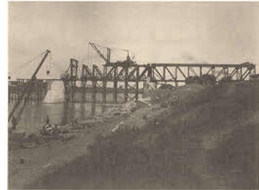
View of the St. Andrews Lock and Dam under construction.
