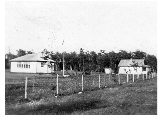
Poplar Park School and Teacherage, built in 1913. This is an excellent example of the kind of one-room school setting in which most children in St. Clements would have experienced.
