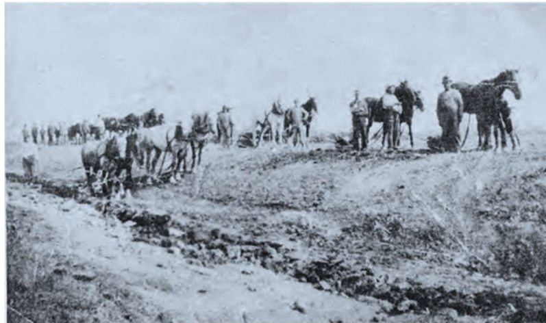
Top: A grader levelling a road bed. Below: A work gang establishing the roadway.
