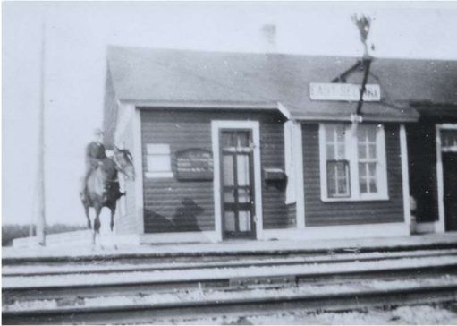
East Selkirk Station.
