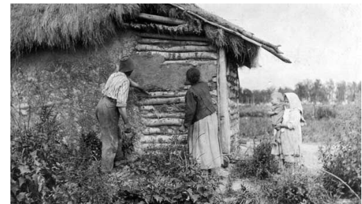
View of a family undertaking the annual re-plastering and whitewashing of the exterior log walls of the farm house.
