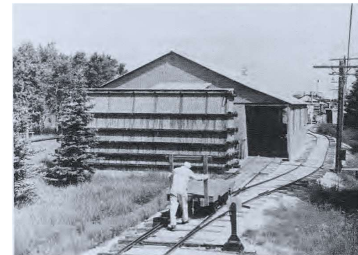
Moving material to a case house at the C.I.L. Explosives Plant.
