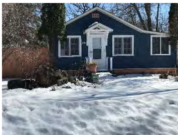
Typical older cabin on Central – note large windows and nice entrance.
