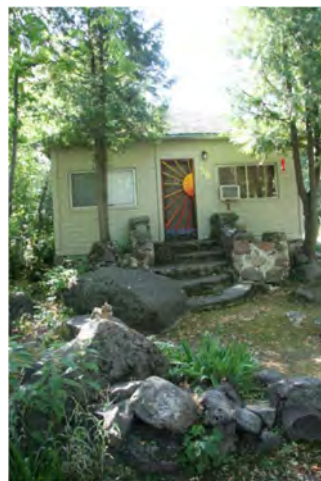
Major example of stone stairs – midpoint of Central – east side.
