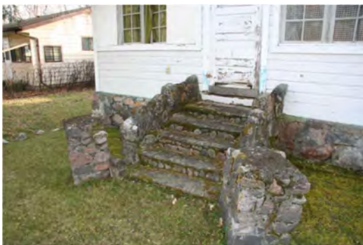
Typical stone stair feature – 6 Poplar.
