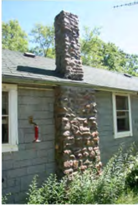
Stone Chimney at Bremont Cottage – 13 Thorncliffe
