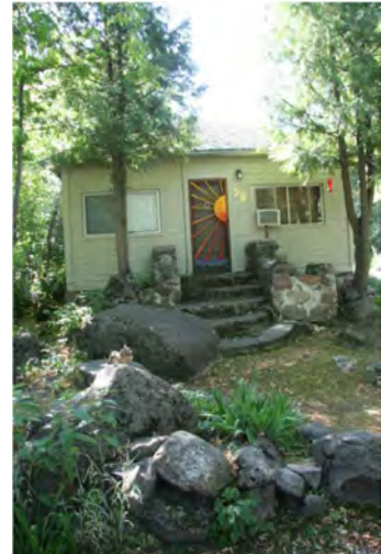
Major example of stone stairs – midpoint of Central – east side.
