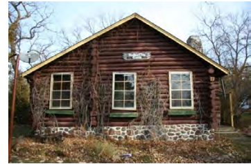
Broken Tree Cottage 77 Grand Marais Blvd N
