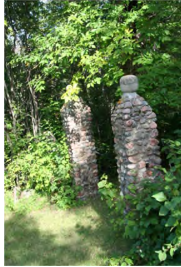
Denardi Fence - posts
