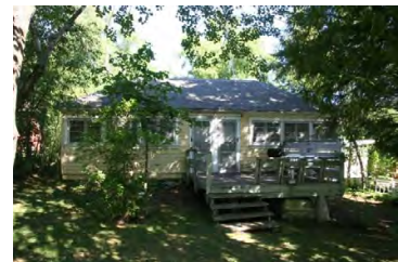
Ashgrove Cottage 31 Central Avenue
