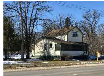
Dairy/Creamery at Grand Beach Road and Glenvale
