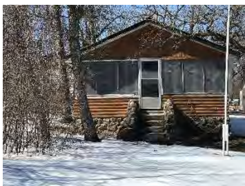
Typical older cabin on Central – note nice stone steps, airy verandah.
