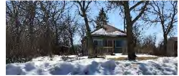
Cabin on Oakdale – note the cottage roof and window arrangement.
