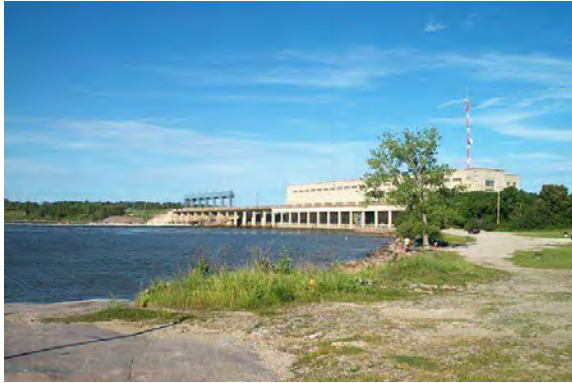
Pine Falls Dam, an important local source of hydro power.
