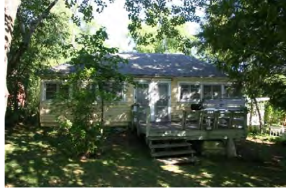
Ashgrove Cottage 31 Central Avenue
