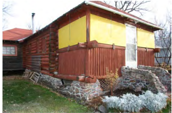
Log Cabin on Grand Marais Blvd N, west of Lakeview - Excellent example of Grand Marais log style – note main building with saddlenotches and porch area with slender vertical pieces for lower wall area.
