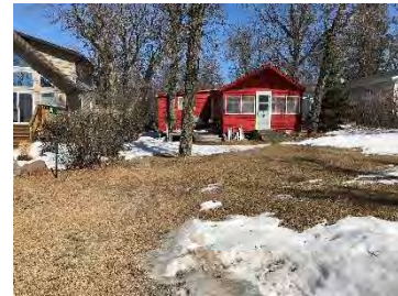
Cabin with interesting roof, Grand Marais Blvd N
