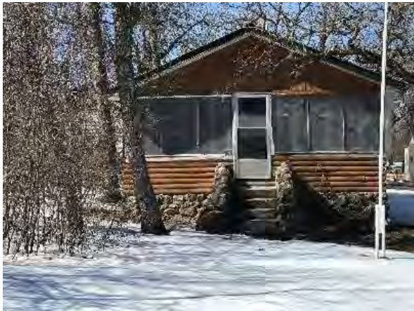
Typical cabin in this area, on Lakeview. Note the “faux” log finish and fine stone foundation and stairs.
