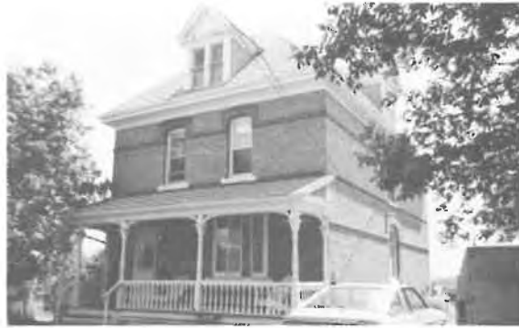
26) 2 1/2 Storey Square Plan House Construction Date: 1911 Location: 478 Eveline Street, Selkirk Present Owner: Mr. G. McLeod Present Use: Occupied Construction: walls - red brick on milled wooden frame roof - asphalt shingles on milled wooden rafters Integrity: Largely unaltered Condition: Good Notes: This building is also discussed on page 120.
