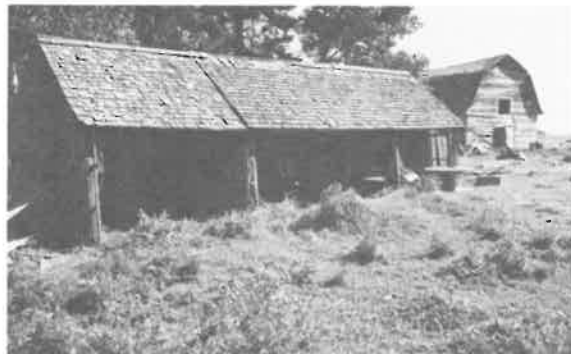
136) Machine Shed Construction Date: ca. 1920 Location: SE 12-16-7E Present Owner: V. Parke Present Use: Abandoned Construction: walls - vertical logs roof - wood shingles on hewn wooden rafters Integrity: Unaltered Condition: Poor
