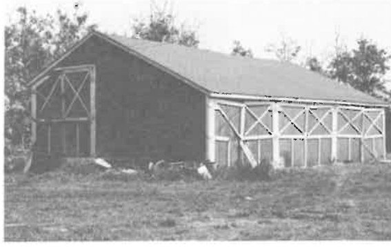
138) Machine Shed Construction Date: 1938 Location: SE 22-16-3E Present Owner: M. Chorney Present Use: Functioning machine shed Construction: walls - horizontal siding on milled wooden frame roof - asphalt shingles on milled wooden rafters Integrity: Unaltered Condition: Good
