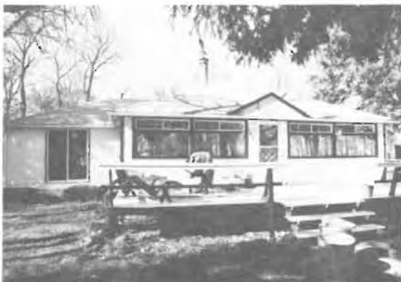
Plate 259. A cottage at Winnipeg Beach altered by external additions, including a deck, and internal winterization.
