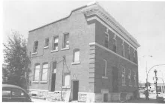
234) Former Custom's Office/Post Office Construction Date: 1905 Location: Main Street, Selkirk Present Owner: Town of Selkirk Present Use: Vacant Construction: walls - red brick on milled wooden frame roof - built-up tar and gravel Integrity: Basically unaltered Condition: Good Notes: This building is also discussed on pages 110-111.
