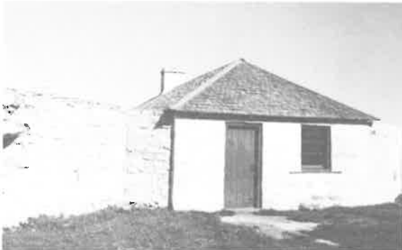
251) Northwest Bastion Construction Date: 1840s Location: Lower Fort Garry National Historic Park Present Owner: Parks Canada Present Use: Display Construction: walls - dressed limestone roof - wood shingles on hewn timber rafters Integrity: The structure has been carefully restored. Condition: Good
