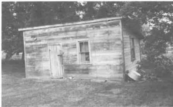
59) Single Storey Shanty Construction Date: ca. 1890 Location: River Lot #199 Present Owner: Mrs. M. Ritchie Present Use: Storage Construction: walls - horizontal siding on milled wooden frame roof - wood shingles on milled wooden rafters Integrity: Largely unaltered Condition: Fair Notes: This building is also discussed on page 58.
