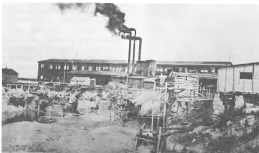
Plate 231. The great stone cutting mill at Garson. (PAM)
