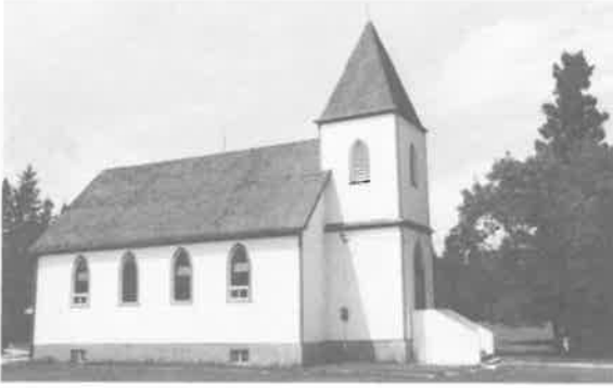
185) Cloverdale United Church Construction Date: 1921 Location: SE 8-14-4E Present Owner: United Church of Canada Present Use: Active Congregation Construction: walls - horizontal siding on milled wooden frame roof - wood shingles on milled wooden rafters Integrity: Largely unaltered Condition: Good Notes: This building is also discussed on pages 94-95.
