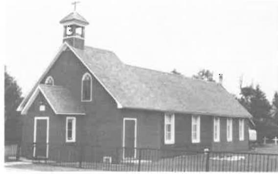
194) St. Anne's Polish Catholic Church Construction Date: 1934 Location: Petersfield Present Owner: Polish Catholic Church of Canada Present Use: Active Congregation Construction: walls - insulbrick siding on milled wooden frame roof - asphalt shingles on milled wooden rafters Integrity: Largely unaltered Condition: Good Notes: This building is also discussed on page 127.
