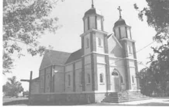
202) Ukrainian Catholic Church Construction Date: 1951 Location: East Selkirk Present Owner: Ukrainian Catholic Church of Canada Present Use: Active Congregation Construction: walls - stucco veneer on milled wooden frame roof - asphalt shingles on milled wooden rafters Integrity: Largely unaltered Condition: Good Notes: This building is also discussed on page 122.
