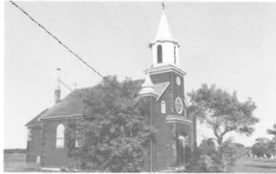
198) Sacred Heart Chapel, Victoria Park Construction Date: 1937 Location: River Lot #70 Present Owner: Present Use: Vacant Construction: walls - insulbrick siding on milled wooden frame roof - wood shingles on milled wooden rafters Integrity: Largely unaltered Condition: Poor Notes: This building has been dismantled and the hall section used as a private residence.
