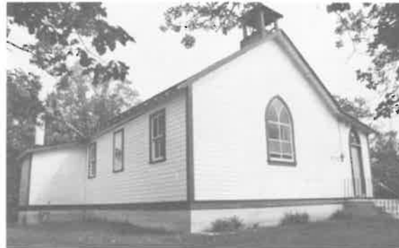
180) MacKenzie Presbyterian Church Construction Date: 1922 Location: River Lot #120 Present Owner: Presbyterian Church of Canada Present Use: Active Congregation Construction: walls - horizontal siding on milled wooden frame roof - asphalt shingles on milled wooden rafters Integrity: Largely unaltered Condition: Good
