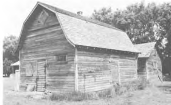
100) Light Wood Frame Barn Construction Date: 1912 Location: River Lot #261 Present Owner: Mr. Henry Semenchuk Present Use: Storage Construction: walls - horizontal siding on milled wooden frame roof - wood shingles on milled wooden rafters Integrity: Unaltered Condition: Good
