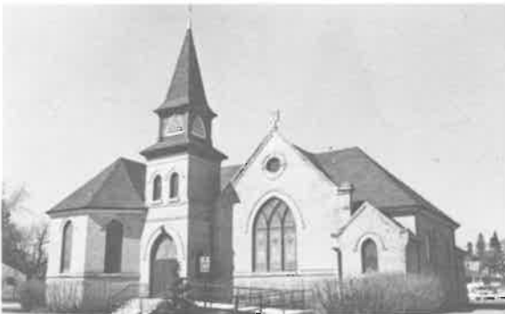
179) Knox Presbyterian Church Construction Date: 1904 Location: Eveline Street, Selkirk Present Owner: Presbyterian Church of Canada Present Use: Active Congregation Construction: walls - buff brick on wood frame roof - asphalt shingles on milled wooden rafters Integrity: Largely unaltered Condition: Good Notes: This building is also discussed on pages 115 and 117.
