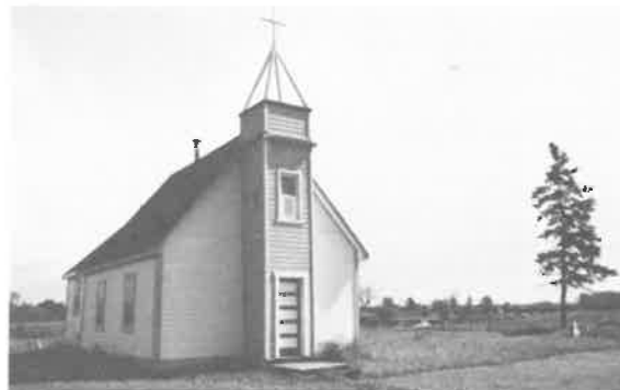
188) Scaterbury Church Construction Date: ca. 1920 Location: River Lot #16 Present Owner: Roman Catholic Church of Canada Present Use: Active Congregation Construction: walls - horizontal siding on milled wooden frame roof - asphalt shingles on milled wooden rafters Integrity: Largely unaltered Condition: Fair
