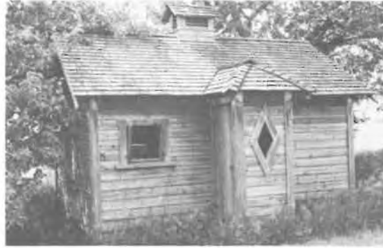
162) Outhouse Construction Date: ca. 1920 Location: Present Owner: Present Use: Vacant Construction: walls - horizontal siding on milled wooden frame roof - wood shingles on milled wooden rafters Integrity: Unaltered Condition: Good
