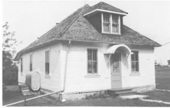
82) 1 1/2 Storey Cottage Construction Date: 1929 Location: River Lot #242 Present Owner: Mrs. Zybyluk Present Use: Occupied Construction: walls - horizontal siding on milled wooden frame roof - wood shingles on milled wooden rafters Integrity: Largely unaltered Condition: Good
