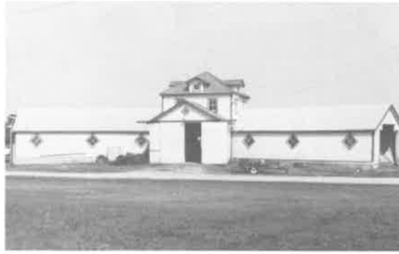
146) Bunkhouse/Machine Shed Construction Date: ca. 1925 Location: NE 2-16-3E Present Owner: C.P. Kollar Present Use: Storage Construction: walls - horizontal siding on milled wooden frame roof - wood shingles on milled wooden rafters Integrity: The attached wings have been altered to accommodate larger machinery Condition: Good Notes: This building is also discussed on page 74.
