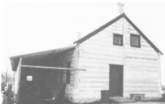
244) Farm Manager's House Construction Date: 1830's Location: Lower Fort Garry National Historic Park Present Owner: Parks Canada Present Use: Display Construction: walls - Red River framed logs roof - wood shingles on hewn timber rafters Integrity: The building has been carefully restored. Condition: Good
