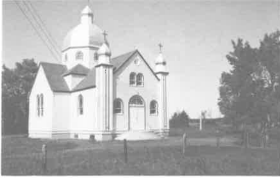
201) St. Peter & St. Paul Ukrainian Catholic Church Construction Date: ca. 1930 Location: SE 19-16-8E Present Owner: Ukrainian Catholic Church of Canada Present Use: Active Congregation Construction: walls - horizontal siding on milled wooden frame roof - asphalt shingles on milled wooden rafters Integrity: Largely unaltered Condition: Good
