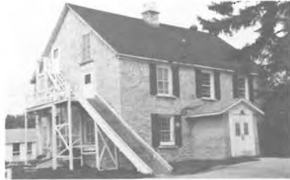
38) St. Peter's Dynevor Indian Hospital Construction Date: 1862-65 Location: River Lot #40 Present Owner: St. John's Cathedral Boy's School Present Use: Administrative Offices Construction: walls - fieldstone roof - asphalt shingles on cut timbers Integrity: The interior has been altered Condition: Fair Notes: This building is also discussed on pages 40-42.
