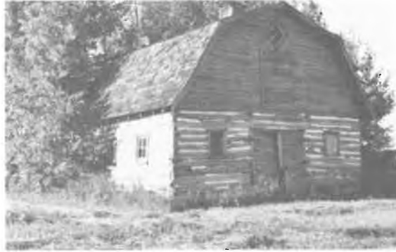
106) Log Barn Construction Date: ca. 1920 Location: SW 34-17-3E Present Owner: Mr. Huminicki Present Use: Storage Construction: walls - dovetailed logs roof - wood shingles on milled wooden rafters Integrity: Unaltered Condition: Fair
