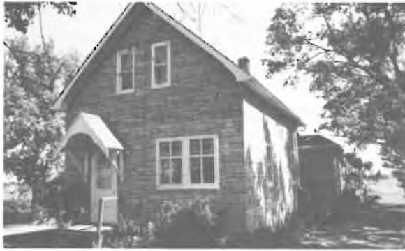
Plate 226. Wood frame house in East Selkirk.
