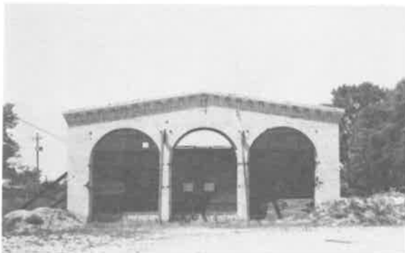
235) Rail Car Garage Construction Date: Location: Eveline Street, Selkirk Present Owner: Present Use: Church Construction: walls - buff brick cavity wall roof - non-existent Integrity: The roof has been removed and the walls are precariously supported Condition: Fair Notes: The building has recently been renovated to accommodate a church.
