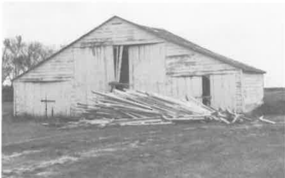
135) Machine Shed Construction Date: ca. 1910 Location: River Lot #120 Present Owner: Province of Manitoba Present Use: Vacant Construction: walls - horizontal siding with milled wooden frame roof - wood shingles on milled wooden rafters Integrity: Unaltered Condition: Poor Notes: The large central doors accommodated a threshing machine
