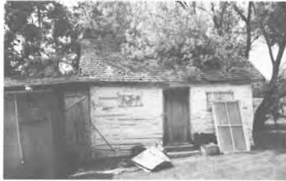
98) Log Barn Construction Date: ca. 1910 Location: River Lot #264 Present Owner: Henry Semenchuk Present Use: Storage Construction: walls - dovetailed squared logs roof - wood shingles on hewn wooden rafters Integrity: Largely unaltered Condition: Fair Notes: This building is also discussed on page 64.
