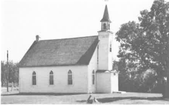
173) St. James Anglican Church Construction Date: 1912 Location: NE 32-15-6E Present Owner: Anglican Church of Canada Present Use: Active Congregation Construction: walls - horizontal siding on milled wooden frame roof - asphalt shingles on milled wooden rafters Integrity: Largely unaltered floorplan Condition: Good Notes: This building is also discussed on pages 93-94.
