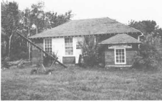
221) Brookside School Construction Date: ca. 1925 Location: SE 11-14-5E Present Owner: W. Jacyk Present Use: Storage Construction: walls - insulbrick veneer on milled wooden frame roof - asphalt shingles on milled wooden rafters Integrity: Unaltered Condition: Good
