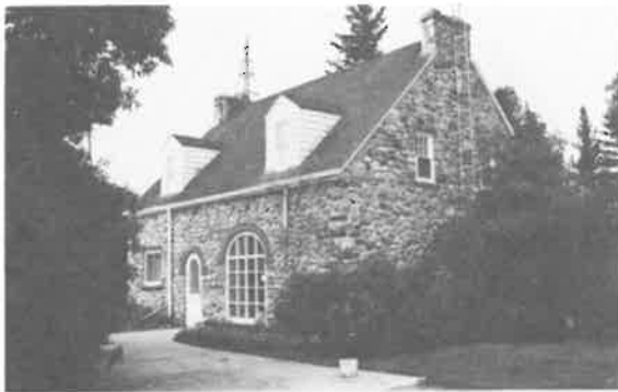
87) 1 1/2 Storey Stone House Construction Date: 1939-41 Location: NW 1-14-5E Present Owner: Mr. W. Buchanan Present Use: Occupied Construction: walls - roof - wood shingles on milled wooden rafters Integrity: Largely unaltered Condition: Good
