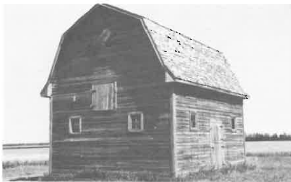
111) Small Light Wood Frame Barn Construction Date: ca. 1925 Location: SW 21-15-6E Present Owner: Present Use: Storage Construction: walls - horizontal siding on milled wooden frame roof - wood shingles on milled wooden rafters Integrity: Unaltered Condition: Good
