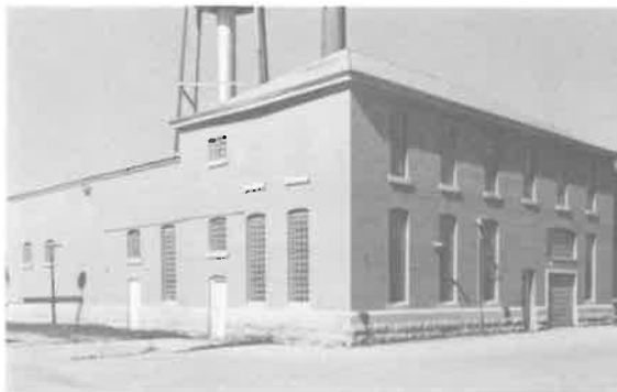
242) Old Power House Construction Date: 1921 Location: Selkirk Mental Health Centre Present Owner: Selkirk Mental Health Centre Construction: walls - brick veneer on milled wooden frame roof - built-up roofing Integrity: Some window openings have been bricked in. Condition: Good
