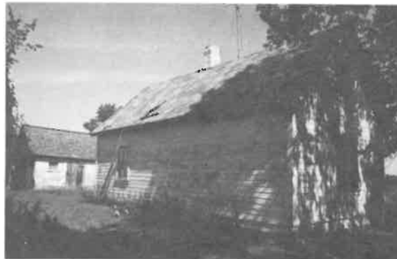
Plate 225. Log house in East Selkirk.
