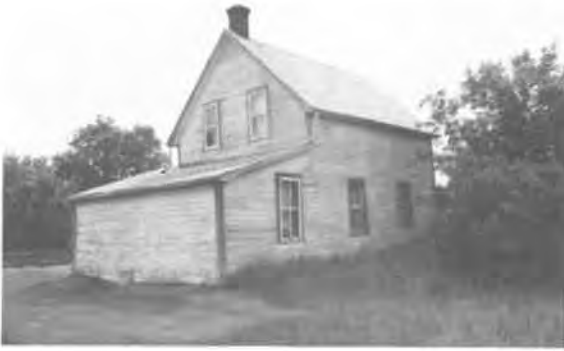
65) 1 1/2 Storey Side Hall House Construction Date: ca. 1910 Location: River Lot #121 Present Owner: A. MacArthur Present Use: Summer occupancy Construction: walls - horizontal siding on milled wooden frame roof - asphalt shingles on milled wooden rafters Integrity: Unaltered floorplan Condition: Good Notes: This building is also discussed on pages 56-58.
