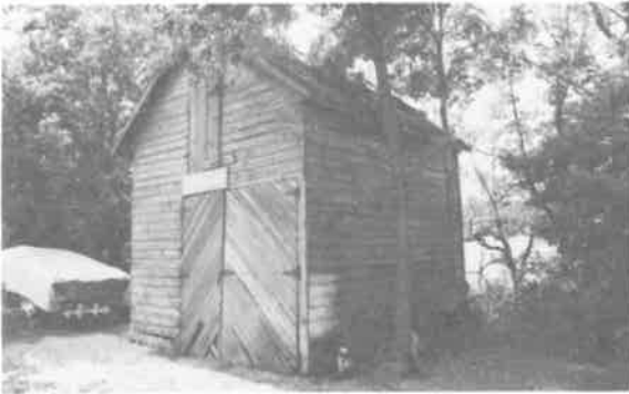
139) Garage Construction Date: ca. 1910 Location: River Lot #255 Present Owner: M. Nebozenko Present Use: Storage Construction: walls - horizontal siding on milled wooden frame roof - wood shingles on milled wooden rafters Integrity: Unaltered Condition: Good Notes: The upper level was used for miscellaneous storage.
