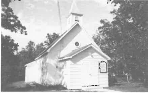
197) St. Joseph's Polish Catholic Church Construction Date: ca. 1920 Location: Libau Present Owner: Polish Catholic Church of Canada Present Use: Active Congregation Construction: walls - aluminum siding on milled wooden frame roof - asphalt shingles on milled wooden rafters Integrity: Largely unaltered Condition: Good
