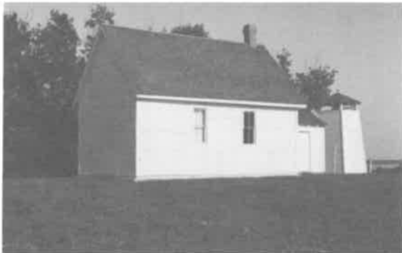
199) Holy Rosary Polish Catholic Church Construction Date: ca. 1910 Location: SE 34-17-3E Present Owner: Polish Catholic Church of Canada Present Use: Occasional service Construction: walls - horizontal siding on milled wooden frame roof - asphalt shingles on milled wooden rafters Integrity: Unaltered Condition: Good
