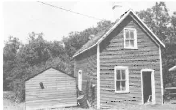
60) 1 1/2 Storey Side Hall House Construction Date: ca. 1890 Location: SW 12-14-3E Present Owner: Mr. Dewar Present Use: Storage Construction: walls - horizontal siding on milled wooden frame roof - wood shingles on milled wooden rafters Integrity: The interior has been altered Condition: Fair
