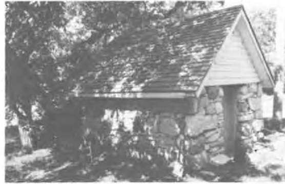
158) Milk House Construction Date: Ca. 1880 Location: River Lot #10 Present Owner: Mrs. Larter Present Use: Storage Construction: walls - solid fieldstone roof - wood shingles on milled wooden rafters Integrity: Unaltered Condition: Good Notes: This building is also discussed on page 76.
