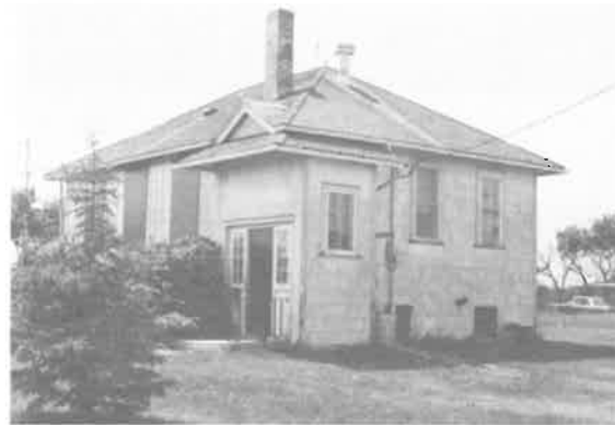
Plate 178. An interesting alternative to Hooper's designs which appeared occasionally in the planning area (here at NE14-15-3E), shifted the entrance to one side and drew it out into a sort of corner tower.
