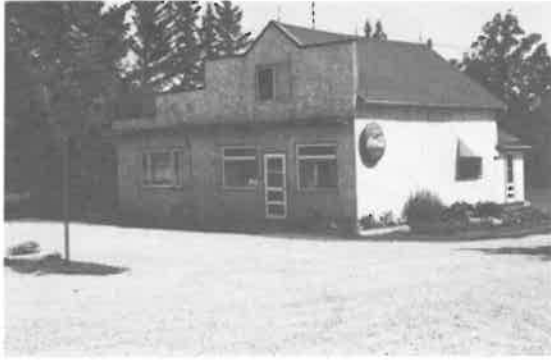
229) General Store Construction Date: ca. 1920 Location: NW 18-16-8E Present Owner: Present Use: Vacant Construction: walls - stucco veneer on milled wooden frame roof - asphalt shingles on milled wooden rafters Integrity: Unaltered Condition: Good
