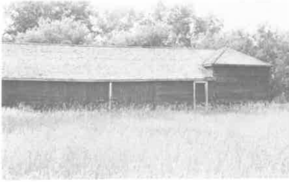
137) Machine Shed Construction Date: ca. 1910 Location: SE 22-16-3E Present Owner: A. Dalman Present Use: Abandoned Construction: walls - horizontal siding on milled wooden frame roof - wood shingles on milled wooden rafters Integrity: Unaltered Condition: Poor
