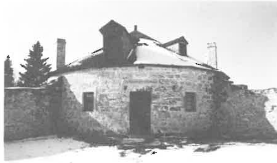
250) Southwest Bastion Construction Date: 1840s Location: Lower Fort Garry National Historic Park Present Owner: Parks Canada Present Use: Display Construction: walls - dressed limestone roof - wood shingles on hewn timber rafters Integrity: The structure has been carefully restored. Condition: Good
