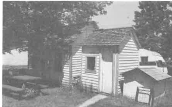
156) Summer Kitchen Construction Date: ca.1915 Location: 423 Sinclair Avenue, Selkirk Present Owner: Mrs. L. Morriseau Present Use: Storage Construction: walls - horizontal siding on milled wooden frame roof - wood shingles on milled wooden rafters Integrity: Unaltered Condition: Good
