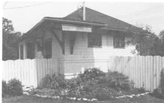
236) East Selkirk Rail Station Construction Date: Location: Present Owner: Mr. R. Andryo Present Use: Workshop Construction: walls - horizontal siding on milled wooden frame roof - asphalt shingles on milled wooden rafters Integrity: The interior has been much altered for its present function Condition: Fair
