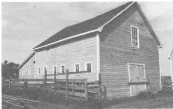
103) Large Light Wood Frame Barn Construction Date: 1915 Location: SE 1-15-4E Present Owner: Mr. Macklin Present Use: Functioning Barn Construction: walls - horizontal siding on milled wooden frame roof - wood shingles on milled wooden rafters Integrity: Unaltered Condition: Good
