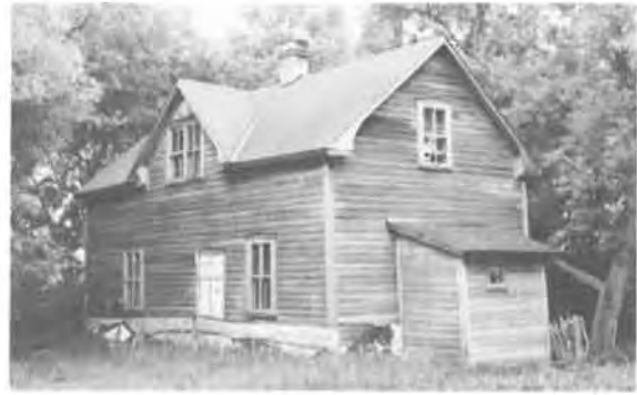
78) 1 1/2 Storey Central Gable House Construction Date: ca. 1890 Location: NW 36-17-3E Present Owner: Mr. N. Swirski Present Use: Occupied Construction: walls - horizontal siding on milled wooden frame roof - asphalt shingles on milled wooden rafters Integrity: Largely unaltered Condition: Fair
