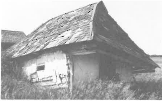
153) Summer Kitchen Construction Date: ca.1900 Location: River Lot #90 Present Owner: Present Use: Abandoned Construction: walls - Plaster cover on dovetailed logs roof - wood shingles on milled wooden rafters Integrity: Unaltered Condition: Poor - the structure is collapsing on the north side
