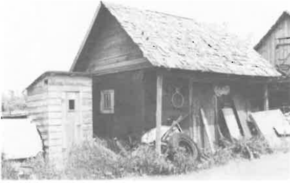
145) Workshop Construction Date: 1932 Location: River Lot #226 Present Owner: W.R. Kozak Present Use: Storage Construction: walls - dovetailed logs roof - wood shingles on milled wooden rafters Integrity: Unaltered Condition: Fair
