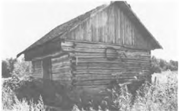
128) Log Granary Construction Date: ca. 1915 Location: SE 19-14-6E Present Owner: Mr. A. Caravan Present Use: Storage Construction: walls - dovetailed logs roof - wooden shingles on milled wooden rafters Integrity: Unaltered Condition: Good
