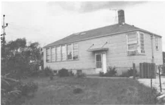
223) Earl Grey School Construction Date: ca. 1925 Location: SW 36-13-3E Present Owner: L. LeBlanc Present Use: Residence Construction: walls - wood shingles on milled wooden frame roof - asphalt shingles on milled wooden rafters Integrity: The interior has undergone renovations for its present function Condition: Good Notes: This building is also discussed on page 104.
