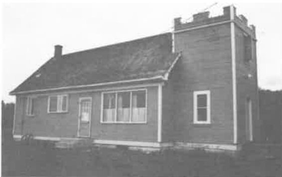
187) MacBeth Church Construction Date: 1932 Location: SE 25-13-5E Present Owner: Present Use: Residence Construction: walls - horizontal siding on milled wooden frame roof - asphalt shingles on milled wooden rafters Integrity: The building has been moved and much altered to fulfill its present function. Condition: Good
