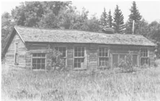
148) Chicken Coop Construction Date: ca. 1920 Location: SE 22-16-3E Present Owner: A. Dalman Present Use: Abandoned Construction: walls - horizontal siding on milled wooden frame roof - wood shingles on milled wooden rafters Integrity: Unaltered Condition: Poor Notes: This building is also discussed on page 75.
