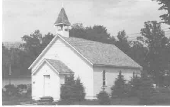
178) St. George's Anglican Church Construction Date: 1938 Location: St. John's Boy's School/River Lot #41 Present Owner: St. John's Cathedral Boy's School Present Use: School Use Construction: walls - horizontal siding on milled wooden frame roof - asphalt shingles on milled wooden rafters Integrity: The church has been moved onto its present site. Condition: Good
