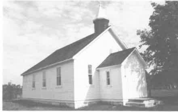
210) Libau Lutheran Church Construction Date: ca. 1920 Location: Libau Present Owner: Lutheran Church of Canada Present Use: Active Congregation Construction: walls - horizontal siding on milled wooden frame roof - wood shingles on milled wooden rafters Integrity: Largely unaltered Condition: Good Notes: This building is also discussed on page 128.
