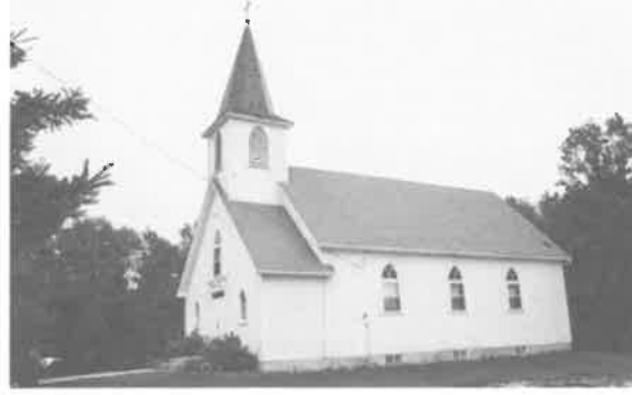
190) St. John's Evangelical Lutheran Church Construction Date: ca. 1920 Location: SW 19-15-8E Present Owner: Lutheran Church of Canada Present Use: Active Congregation Construction: walls - horizontal siding on milled wooden frame roof - asphalt shingles on milled wooden rafters Integrity: Largely unaltered Condition: Good
