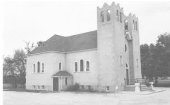
196) St. Margaret's Roman Catholic Church, Little Britain Construction Date: 1943 Location: River Lot #120 Present Owner: Roman Catholic Church of Canada Present Use: Active Congregation Construction: walls - stucco veneer on milled wooden frame roof - asphalt shingles on milled wooden rafters Integrity: Largely unaltered Condition: Good
