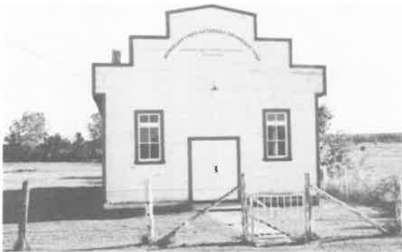
211) Poplar Park Ukrainian Greek Catholic Parish Hall Construction Date: 1923 Location: NE 34-15-6E Present Owner: Ukrainian Greek Catholic Church of Canada Present Use: Active Hall Construction: walls - horizontal siding on milled wooden frame roof - asphalt shingles on milled wooden rafters Integrity: Unaltered Condition: Good Notes: This building is also discussed on page 101.
