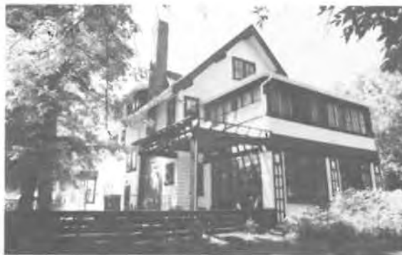
92) 2 1/2 Storey House Construction Date: 1919 Location: River Lot #114 Present Owner: Ms. Schadek Present Use: Occupied Construction: walls - horizontal siding on milled wooden frame roof - asphalt shingles on milled wooden rafters Integrity: Largely unaltered Condition: Good
