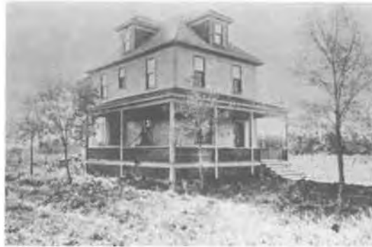
Plate 219. The former Smith house on Eveline Street, built in 1916, has one of the earliest poured concrete basements in Selkirk.
