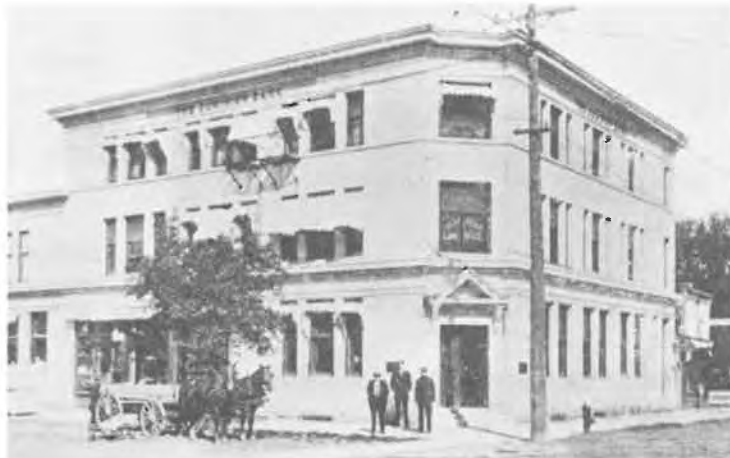
Plate 203. The Merchant's Hotel has been covered with stucco about the main floor, eliminating many of the building's original and interesting features. (PAM)
