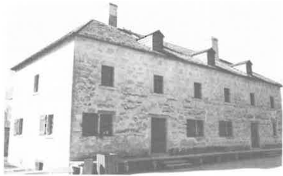
246) Fur House Construction Date: 1831 Location: Lower Fort Garry National Historic Park Present Owner: Parks Canada Present Use: Display Construction: walls - dressed limestone roof - wood shingles on hewn timber rafters Integrity: The building has been carefully restored Condition: Good Notes: This building is also discussed on page 33.
