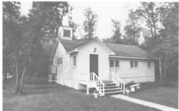
176) All Saints Anglican Church Construction Date: 1922 Location: Whyteford Present Owner: Anglican Church of Canada Present Use: Active Congregation Construction: walls - horizontal siding on milled wooden frame roof - asphalt shingles on milled wooden rafters Integrity: Largely unaltered Condition: Good
