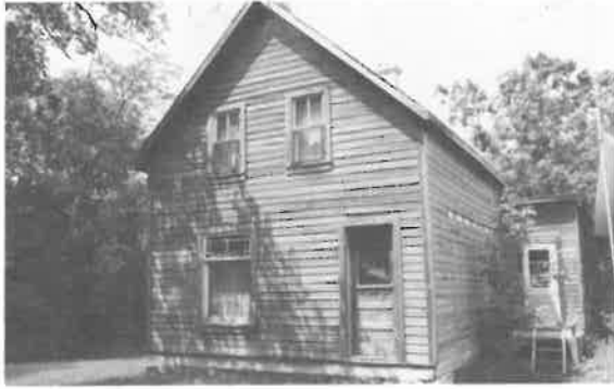
61) 1 1/2 Storey Side Hall House Construction Date: ca. 1905 Location: River Lot #255 Present Owner: S. Michaelson Present Use: Vacant Construction: walls - horizontal siding on milled wooden frame roof - asphalt shingles on milled wooden rafters Integrity: Largely unaltered Condition: Fair
