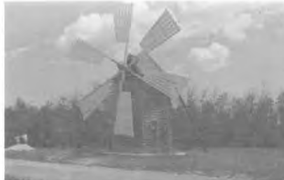
164) Windmill Construction Date: ca. 1910 Location: Winnipeg Beach Ukrainian Heritage Museum Present Owner: Winnipeg Beach Ukrainian Heritage Museum Present Use: Display Construction: Wood shingles on wooden frame on roughly hewn logs Integrity: The building has been moved to its present site and numerous changes have been made to the interior. The sails are of recent construction. Condition: Good Notes: This building is also discussed on pages 90-91.
