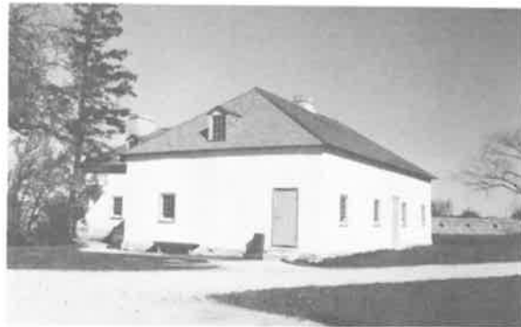
248) Men's House Construction Date: 1850s Location: Lower Fort Garry National Historic Park Present Owner: Parks Canada Present Use: Display Construction: walls - dressed limestone roof - wooden shingles on hewn timber rafters Integrity: The building has been carefully restored Condition: Good
