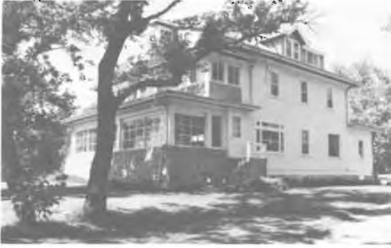
89) 2 1/2 Storey Square Plan House Construction Date: 1912 Location: River Lot #17 Present Owner: Mrs. Fox Present Use: Occupied Construction: walls - horizontal siding on milled wooden frame roof - asphalt shingles on milled wooden rafters Integrity: Largely unaltered Condition: Good Notes: This building is also discussed on pages 61-63.
