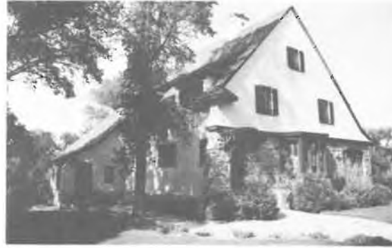
90) 2 1/2 Storey House Construction Date: 1918 Location: River Lots #117-119 Present Owner: Dr. Olafson Present Use: Occupied Construction: walls - stone and stucco veneer on milled wooden frame roof - asphalt shingles on milled wooden rafters Integrity: Unaltered floorplan Condition: Good Notes: This building stands on the site of the original Hawthorne Lodge, discussed on page 29.
