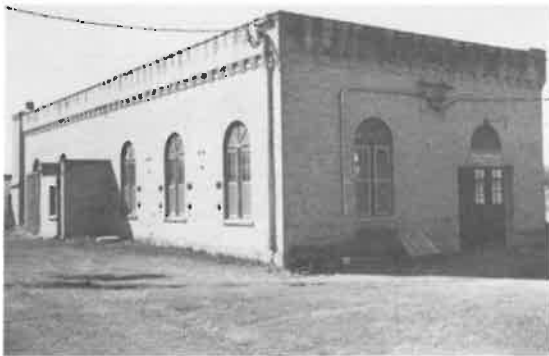
231) Power Station Construction Date: 1910 Location: Lockport Present Owner: Department of Public Works Present Use: Functioning Power Station Construction: walls - buff brick veneer on milled wooden frame roof - built up roofing Integrity: Largely unaltered Condition: Good Notes: This building is also discussed on page 129.
