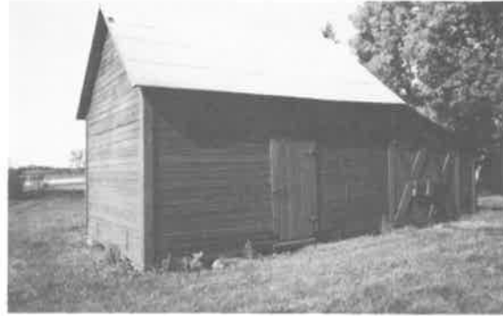
130) Granary Construction Date: ca. 1930 Location: SW 27-15-6E Present Owner: Present Use: Storage Construction: walls - horizontal siding on milled wooden frame roof - wood shingles on milled wooden rafters Integrity: Unaltered Condition: Good
