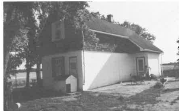
64) 1 1/2 Storey Side Hall House Construction Date: ca. 1910 Location: NW 24-15-6E Present Owner: Mr. C. Horbady Present Use: Occupied Construction: walls - stucco and shingle veneer on milled wooden frame roof - asphalt shingles on milled wooden rafters Integrity: Largely unaltered Condition: Good
