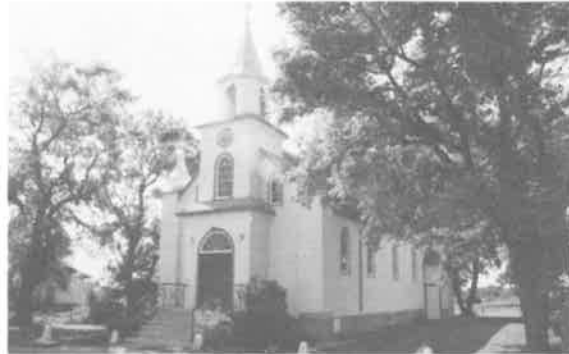
192) St. Stanislaus Roman Catholic Church Construction Date: ca. 1910 Location: East Selkirk Present Owner: Roman Catholic Church of Canada Present Use: Active Congregation Construction: walls - stucco veneer on milled wooden frame roof - asphalt shingles on milled wooden rafters Integrity: Largely unaltered Condition: Good Notes: This building is also discussed on page 122.
