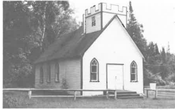
174) St. Luke's Anglican Church, Balsam Bay Construction Date: ca. 1920 Location: SW 28-17-7E Present Owner: Anglican Church of Canada Present Use: Active Congregation Construction: walls - squared dovetailed logs roof - asphalt shingles on milled wooden rafters Integrity: Largely unaltered Condition: Good
