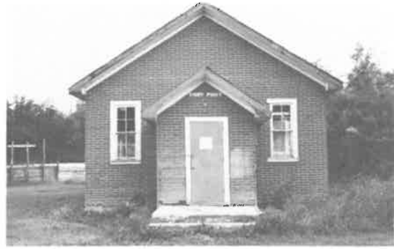
222) Stony Point School Construction Date: ca. 1925 Location: SE 6-17-7E Present Owner: R.M. of St. Clements Present Use: Vacant Construction: walls - insulbrick veneer on milled wooden frame roof - asphalt shingles on milled wooden rafters Integrity: Unaltered Condition: Poor
