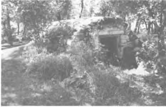
161) Root Cellar Construction Date: ca. 1920 Location: SE 2-13-5E Present Owner: J. Letecki Present Use: Storage Construction: walls - fieldstone barrel vault roof - fieldstone, covered with sod Integrity: Unaltered Condition: Good Notes: This building is also discussed on page 75.
