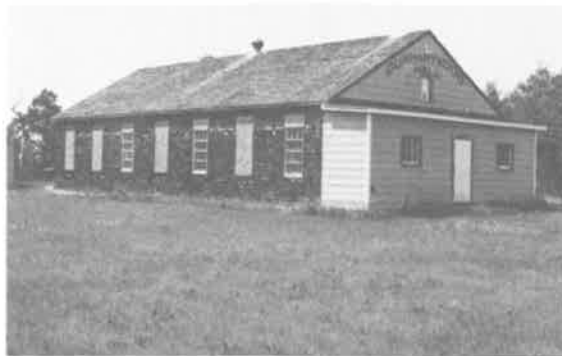
212) Dunhartwood Hall Construction Date: ca. 1940 Location: SE 36-15-3E Present Owner: Present Use: Occasional Use Construction: walls - wood shingles on milled wooden frame roof - wood shingles on milled wooden rafters Integrity: A porch addition of recent construction mars the facade. Condition: Good Notes: This building is also discussed on page 101.
