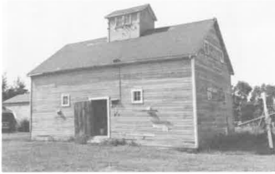
133) Elevator Construction Date: 1915 Location: SE 1-15-4E Present Owner: Mr. Macklin Present Use: Functioning Elevator Construction: walls - horizontal siding on milled wooden frame roof - asphalt shingles on milled wooden rafters Integrity: Unaltered Condition: Good Notes: this building is also discussed on pages 72-73.
