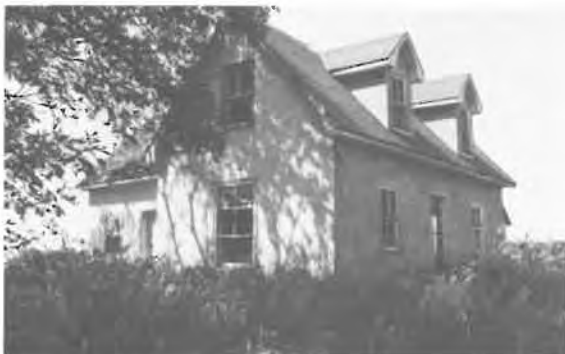
79) 1 1/2 Storey Central Plan House Construction Date: ca. 1920 Location: SE 33-15-6E Present Owner: S. Myslawchuk Present Use: Vacant Construction: walls - stucco veneer on milled wooden frame roof - wood shingles on milled wooden rafters Integrity: Largely unaltered Condition: Poor
