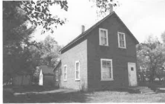
62) 1 1/2 Storey Side Hall House Construction Date: ca. 1905 Location: River Lot #97 Present Owner: M. Clark Present Use: Occupied Construction: walls - insulbrick siding on milled wooden frame roof - wood shingles on milled wooden rafters Integrity: Largely unaltered Condition: Fair
