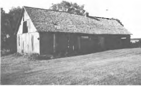
97) Heavy Wood Frame Barn Construction Date: ca. 1910 Location: NW 24-15-6E Present Owner: Mr. C. Horbady Present Use: Storage Construction: walls - horizontal and vertical siding on heavy wood frame roof - wood shingles on milled wooden rafters Integrity: Unaltered Condition: Fair
