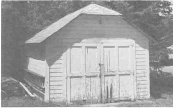
140) Garage Construction Date: 1900 Location: 149 Eveline Street, Selkirk Present Owner: Mrs. Lulashyk Present Use: Functioning garage Construction: walls - horizontal siding on milled wooden frame roof - asphalt shingles on milled wooden rafters Integrity: Unaltered Condition: Fair
