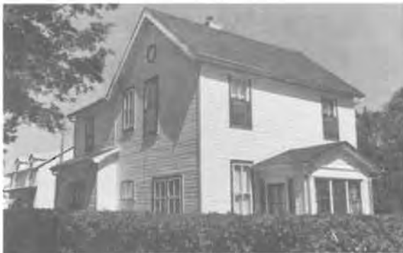
27) 1 1/2 Storey L-Shaped House Construction Date: ca. 1910 Location: 285 Eveline Street, Selkirk Present Owner: Mr. Edward Lennon Present Use: Occupied Construction: walls - horizontal siding on milled wooden frame roof - asphalt shingles on milled wooden rafters Integrity: Largely unaltered Condition: Good
