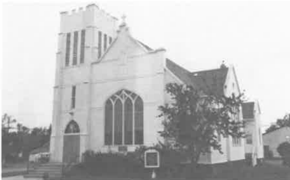
191) Icelandic Evangelical Lutheran Church Construction Date: 1924 Location: Clandeboye Avenue, Selkirk Present Owner: Lutheran Church of Canada Present Use: Active Congregation Construction: walls - horizontal siding on milled wooden frame roof - asphalt shingles on milled wooden rafters Integrity: Largely unaltered Condition: Good Notes: This building is also discussed on page 117.
