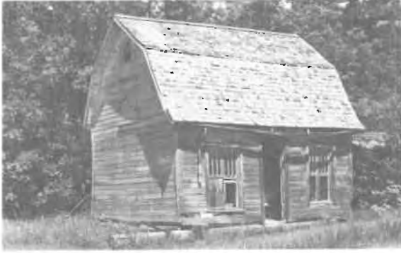
105) Small Light Wood Frame Barn Construction Date: ca. 1915 Location: River Lots 89 and 90 Present Owner: Mr. Kartzmark Present Use: Storage Construction: walls - horizontal siding on milled wooden frame roof - wood shingles on milled wooden rafters Integrity: The interior has been altered for its later function as a residence Condition: Fair
