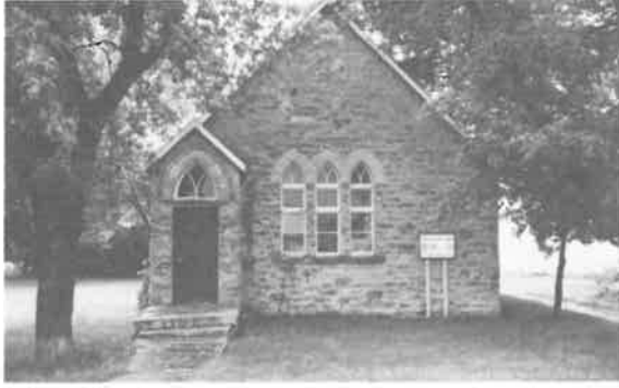
189) Gerson Mission Church Construction Date: 1919 Location: Gerson Present Owner: Baptist Church of Canada Present Use: Active Congregation Construction: walls - solid fieldstone roof - asphalt shingles on milled wooden rafters Integrity: Largely unaltered Condition: Good Notes: This building is also discussed on page 125.
