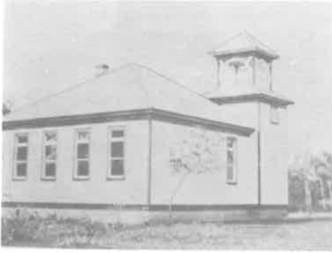
Plate 176. The former Mapleton School had the distinctive offset, detailed tower, square plan and fenestration treatment typical of Hooper's Design No. 3. (From: Beyond the Gates of Lower Fort Garry , p. 78.)
