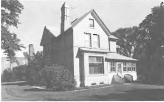
25) 1 1/2 Storey Square Plan House Construction Date: ca. 1890 Location: Selkirk Mental Health Centre Grounds Present Owner: Selkirk Mental Health Centre Present Use: Occupied Construction: walls - buff brick on milled wooden frame roof - asphalt shingles on milled wooden rafters Integrity: Largely unaltered Condition: Good
