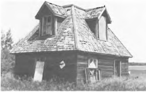
77) 1 1/2 Storey Cottage Construction Date: ca. 1915 Location: NW 19-15-4E Present Owner: J. Hacking Present Use: Vacant Construction: walls - horizontal siding on milled wooden frame roof - wood shingles on milled wooden rafters Integrity: Largely unaltered Condition: Poor
