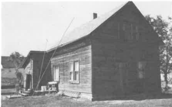
63) 1 1/2 Storey Side Hall House Construction Date: ca. 1910 Location: NE 32-16-8E Present Owner: L. Turner & R. Dick Present Use: Occupied Construction: walls - horizontal siding on milled wooden frame roof - asphalt shingles on milled wooden rafters Integrity: Largely unaltered Condition: Fair
