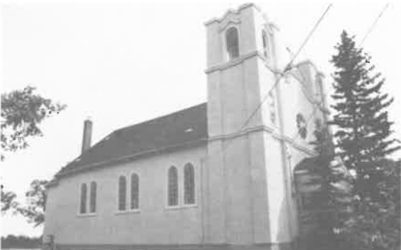
195) Corpus Christi Roman Catholic Church Construction Date: 1940 Location: River Lots 217 & 218 Present Owner: Roman Catholic Church of Canada Present Use: Active Congregation Construction: walls - stucco veneer on milled wooden frame roof - asphalt shingles on milled wooden rafters Integrity: Largely unaltered Condition: Good Notes: This building is also discussed on page 95.
