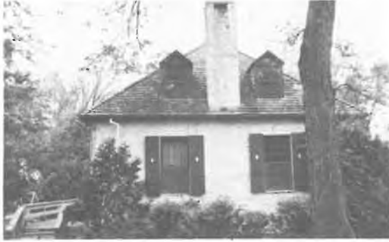
37) Bunn House Construction Date: 1861-64 Location: River Lot #97 Present Owner: The Stewart Brothers Present Use: Summer residence Construction: walls - fieldstone roof - wood shingles on cut timbers Integrity: Unaltered Condition: Good Notes: This building is also discussed on pages 36-38.
