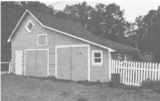
163) Pump House Construction Date: ca. 1915 Location: River Lot #82 Present Owner: Present Use: Storage Construction: walls - horizontal siding on milled wooden frame roof - wood shingles on milled wooden rafters Integrity: Unaltered Condition: Fair
