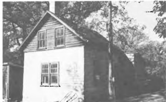
40) Log House Construction Date: ca. 1895 Location: Present Owner: Mrs. West Present Use: Cottage Construction: walls - squared dovetailed logs roof - shingles on milled wooden rafters Integrity: Largely unaltered Condition: Good
