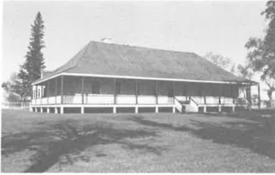
245) Big House Construction Date: 1831 Location: Lower Fort Garry National Historic Park Present Owner: Parks Canada Present Use: Display Construction: walls - dressed limestone roof - wood shingles on hewn timber rafters Integrity: The building has been carefully restored Condition: Good Notes: This building is also discussed on page 32.
