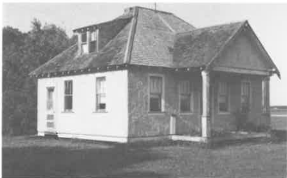
83) 1 1/2 Storey Central Plan House Construction Date: ca. 1930 Location: NE 14-17-3E Present Owner: Mr. V. Nitche Present Use: Storage Construction: walls - stucco veneer on milled wooden frame roof - wood shingles on milled wooden rafters Integrity: Largely unaltered Condition: Good
