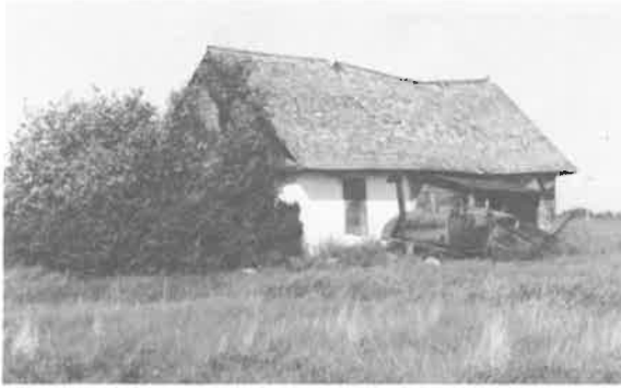
57) Galician Log House Construction Date: ca. 1920 Location: Present Owner: Mr. Sawchuk Present Use: Abandoned Construction: walls - plaster veneer on square dovetailed logs roof - wood shingles on squared logs Integrity: Largely unaltered Condition: Poor
