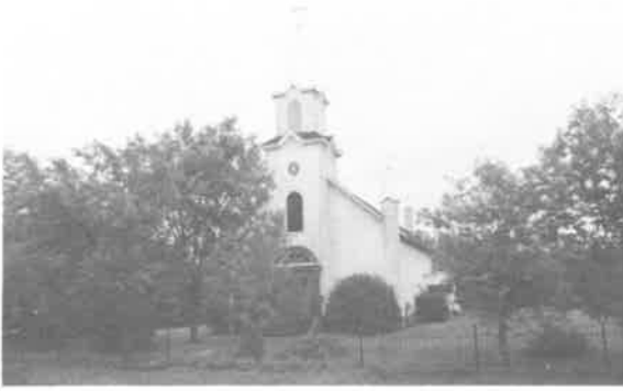
193) Sacred Heart of Jesus Roman Catholic Church Construction Date: ca. 1920 Location: Garson Present Owner: Roman Catholic Church of Canada Present Use: Active Congregation Construction: walls - stucco veneer on milled wooden frame roof - asphalt shingles on milled wooden rafters Integrity: Largely unaltered Condition: Good
