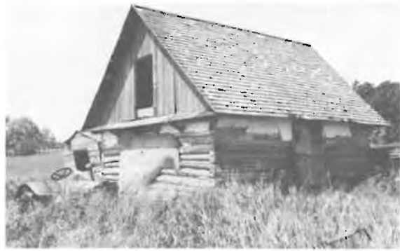
126) Log Granary Construction Date: ca. 1910 Location: Present Owner: Present Use: Vacant Construction: walls - dovetailed logs with plaster cover roof - wood shingles on milled wood rafters Integrity: Unaltered, but plaster is disintegrating Condition: Fair
