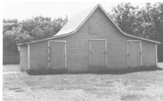
132) Granary Construction Date: ca. 1920 Location: River Lot #71 Present Owner: Present Use: walls - horizontal siding on milled wooden frame roof - wood shingles on milled wooden rafters Integrity: Unaltered Condition: Good Notes: The central section of the building is for grain storage; the projecting wings house crushing equipment and related machinery
