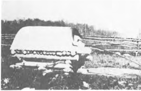
157) Bake Oven Construction Date: c.a. 1920 Location: Winnipeg Beach Ukrainian Heritage Museum Present Owner: Winnipeg Beach Ukrainian Heritage Museum Present Use: Display Construction: Clay and rubble formed into a small vault Integrity: Unaltered Condition: Good Notes: This structure is also discussed on page 89.
