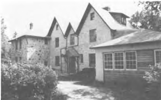
39) Kennedy House Construction Date: 1866-70 Location: River Lot #70 Present Owner: Manitoba Parks Branch Present Use: Tourist Attraction/Tea Room Construction: walls - fieldstone roof - wood shingles on cut timbers Integrity: The interior has been greatly altered and the exterior has been modified. Condition: Good Notes: This building is also discussed on pages 42-43.
