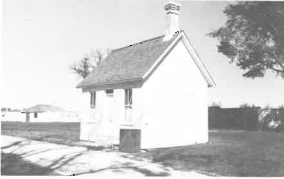
249) Doctor's Office Construction Date: 1885 Location: Lower Fort Garry National Historic Park Present Owner: Parks Canada Present Use: Storage Construction: walls - horizontal siding on milled wooden frame roof - wood shingles on milled wooden rafters Integrity: The building has been carefully restored. Condition: Good
