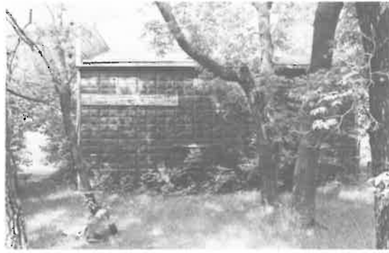
230) General Store Construction Date: ca. 1910 Location: SE 3-15-4E Present Owner: M. Zelyk Present Use: Vacant Construction: walls - pressed tin on milled wooden frame roof - asphalt shingles on milled wooden rafters Integrity: Both interior and exterior have been altered. Condition: Fair
