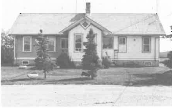
85) Single Storey House Construction Date: 1928 Location: NE 2-16-3E Present Owner: Mr. C.P. Kollar Present Use: Occupied Construction: walls - horizontal siding on milled wooden frame roof - asphalt shingles on milled wooden rafters Integrity: Largely unaltered Condition: Good
