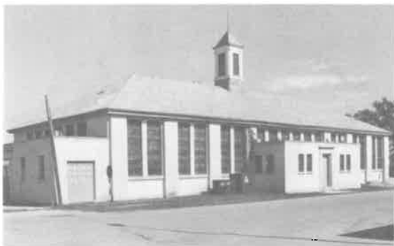
241) Laundry Building Construction Date: 1920 Location: Selkirk Mental Health Centre Present Owner: Selkirk Mental Health Centre Present Use: Laundry facility Construction: walls - stucco veneer on milled wooden frame roof - asphalt shingles Integrity: Largely unaltered Condition: Good
