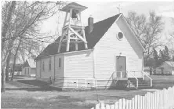
175) St. Bartholomew's Anglican Church Construction Date: 1909 Location: Winnipeg Beach Present Owner: Anglican Church of Canada Present Use: Active Congregation Construction: walls - horizontal siding on milled wooden frame roof - asphalt shingles on milled wooden rafters Integrity: Largely unaltered. Condition: Good Notes: This building is also discussed on pages 133.
