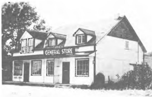
Plate 254. Commercial structure at Grand Marais. (PAM)
