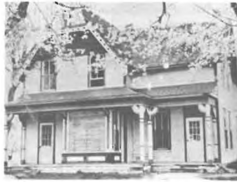
Plate 218. Souter house, Eveline Street. This early photograph shows the original detailing.
