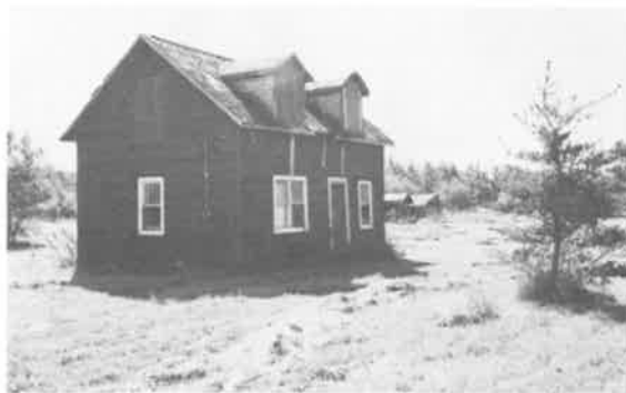
84) 1 1/2 Storey Central Plan House Construction Date: ca. 1930 Location: NE 32-16-7E Present Owner: Mr. A. Hourie Present Use: Vacant Construction: walls - insulbrick veneer on milled wooden frame roof - wood shingles on milled wooden rafters Integrity: Largely unaltered Condition: Poor
