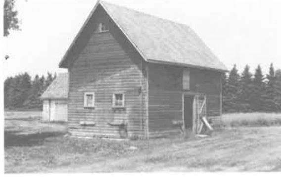
102) Light Wood Frame Stable Construction Date: 1913 Location: NE 15-15-3E Present Owner: Mrs. C.S. Pruden Present Use: Storage Construction: walls - horizontal siding on milled wooden frame roof - wood shingles on milled wooden rafters Integrity: Unaltered Condition: Good Notes: This building is also discussed on pages 65 and 67.
