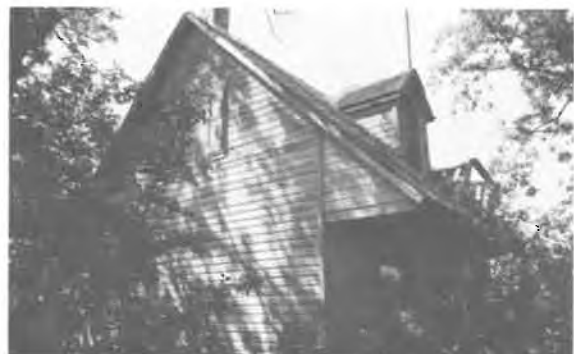
80) 1 1/2 Storey House Construction Date: ca. 1925 Location: NE 9-14-4E Present Owner: J. Clouston Present Use: Vacant Construction: walls - horizontal siding on milled wooden frame roof - wood shingles on milled wooden rafters Integrity: Largely unaltered Condition: Poor
