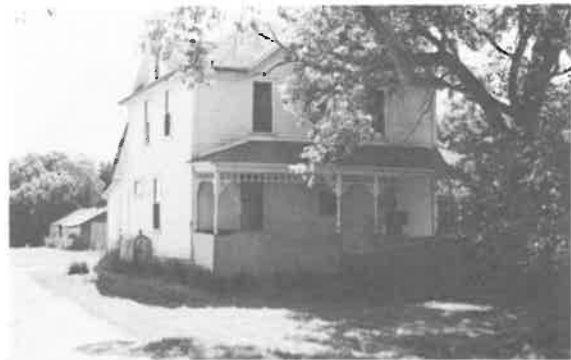
88) 2 1/2 Storey Square Plan House Construction Date: ca. 1910 Location: SW 35-14-4E Present Owner: E. Bracken Present Use: Vacant Construction: walls - horizontal siding on milled wooden frame roof - asphalt shingles on milled wooden rafters Integrity: Largely unaltered Condition: Good Notes: This building is also discussed on page 61.
