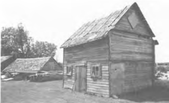
99) Light Wood Frame Stable Construction Date: ca. 1910 Location: River Lot #255 Present Owner: Mr. M. Nebozonko Present Use: Storage Construction: walls - horizontal siding on milled wooden frame roof - wood shingles on milled wooden rafters Integrity: Unaltered Condition: Good
