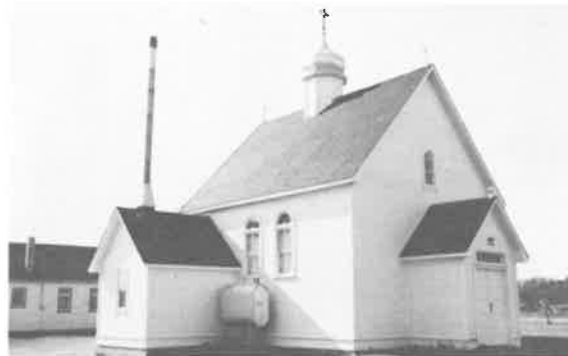
200) St. John the Baptist Ukrainian Catholic Church Construction Date: ca. 1920 Location: NE 34-15-6E Present Owner: Ukrainian Catholic Church of Canada Present Use: Active Congregation Construction: walls - horizontal siding on milled wooden frame roof - asphalt shingles on milled wooden rafters Integrity: Largely unaltered Condition: Good
