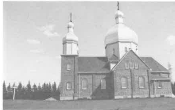
204) Blessed Virgin Mary Ukrainian Catholic Church Construction Date: 1958-60 Location: River Lots 78 & 79 Present Owner: Ukrainian Catholic Church of Canada Present Use: Active Congregation Construction: walls - buff brick on wood frame roof - asphalt shingles on milled wooden rafters Integrity: Unaltered floorplan Condition: Good Notes: This building is also discussed on page 100.
