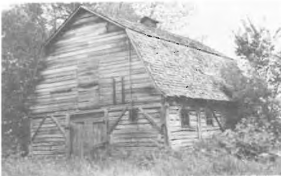
107) Log Barn Construction Date: ca. 1920 Location: NW 35-17-3E Present Owner: Mr. C. Stutsky Present Use: Vacant Construction: walls - Post-and-Sill Logs roof - wood shingles on milled wooden rafters Integrity: Unaltered Condition: Good Notes: Like earlier Ukrainian barns in other areas of the province, this log structure was supported at its corners with diagonal braces.
