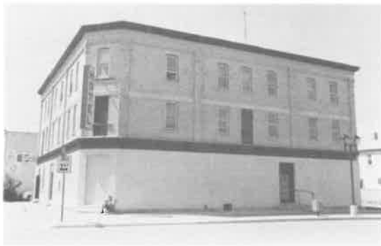
232) Merchant's Hotel Construction Date: 1903 Location: Manitoba & Eveline, Selkirk Present Owner: Verna Konowalchuk Present Use: Functioning Hotel Construction: walls - buff brick on milled wooden frame roof - built-up tar and gravel Integrity: Both interior and exterior have been altered. Condition: Good Notes: This building is also discussed on page 114.
