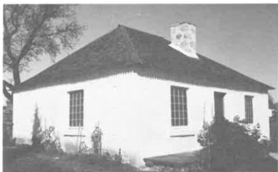
243) Ross Cottage Construction Date: 1840's Location: Lower Fort Garry National Historic Park Present Owner: Parks Canada Present Use: Display Construction: walls - dressed fieldstone roof - wood shingles on hewn timber rafters Integrity: The building has been carefully restored. Condition: Good
