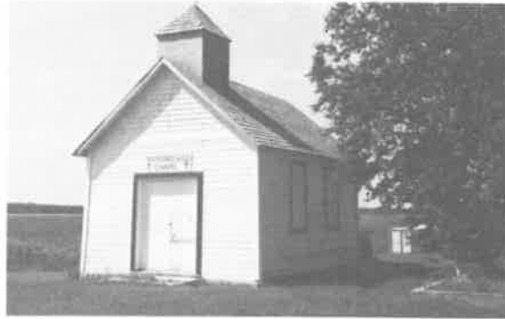
186) Mustard Seed Chapel Construction Date: 1901 Location: SE 34-16-4E Present Owner: Anglican Church of Canada Present Use: Occasional Use Construction: walls - horizontal siding on milled wooden frame roof - wood shingles on milled wooden rafters Integrity: Large unaltered Condition: Good
