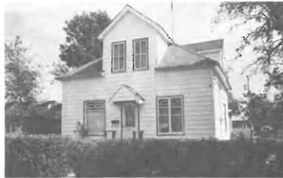
28) 1 1/2 Storey Square Plan House Construction Date: ca. 1900 Location: 517 McLean Avenue, Selkirk Present Owner: Mrs. Kushliak Present Use: Occupied Construction: walls - horizontal siding on milled wooden frame roof - asphalt shingles on milled wooden rafters Integrity: Largely unaltered Condition: Good
