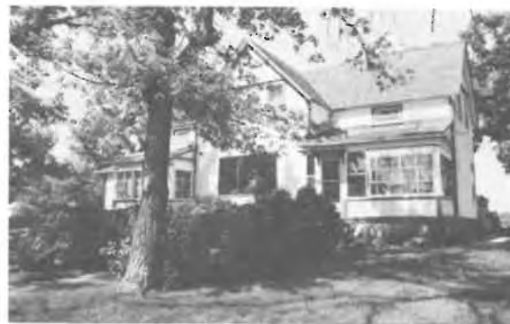
68) 1 1/2 Storey T-shaped House Construction Date: ca. 1890 Location: River Lot #18 Present Owner: Mr. Slyker Present Use: Occupied Construction: walls - horizontal siding on milled wooden frame roof - asphalt shingles on milled wooden rafters Integrity: Only the original kitchen area has been altered Condition: Good
