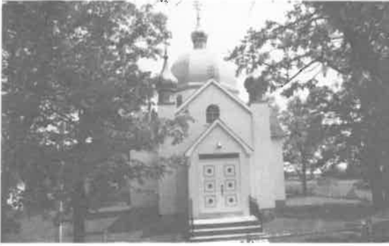
209) St. Nicholas Orthodox Church of Narol Construction Date: 1948 or 1952 Location: River Lot #228 Present Owner: Ukrainian Orthodox Church of Canada Present Use: Active Congregation Construction: wall - stucco veneer on milled wooden frame roof - wood shingles on milled wooden rafters Integrity: Largely unaltered Condition: Good Notes: This building is also discussed on pages 98-99.
