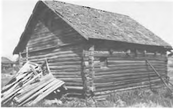
125) Log Granary Construction Date: 1906 Location: SW 18-16-8E Present Owner: Mr. Otto Present Use: Storage Construction: walls - round lap-notched logs roof - wood shingles on milled wood rafters Integrity: Unaltered Condition: Fair
