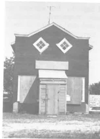
Plate 183. The old Netley Airport Store on Highway No. 9.
