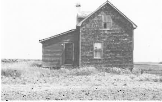
81) 1 1/2 Storey House Construction Date: ca. 1925 Location: SW 23-16-3E Present Owner: R. Penner Present Use: Vacant Construction: walls - wood shingles on milled wooden frame roof - wood shingles on milled wooden rafters Integrity: Largely unaltered Condition: Fair
