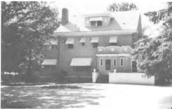
91) 2 1/2 Storey House Construction Date: 1915 Location: River Lot #114 Present Owner: Dr. Robertson Present Use: Occupied Construction: walls - stucco veneer on milled wooden frame roof - asphalt shingles on milled wooden rafters Integrity: Largely unaltered Condition: Good
