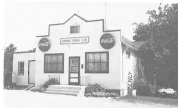
Plate 185. Newman's General Store is cast in stucco, giving it a sleek appearance.
