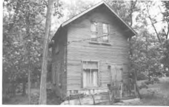
66) 1 1/2 Storey Side Hall House Construction Date: ca. 1915 Location: River Lot #117 Present Owner: Mr. C. Douglas Present Use: Vacant Construction: walls - horizontal siding on milled wooden frame roof - asphalt shingles on milled wooden rafters Integrity: Largely unaltered Condition: Good
