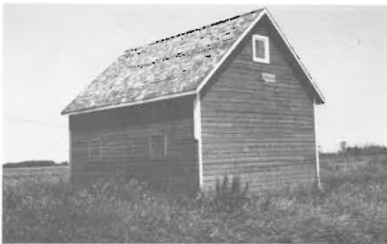
131) Granary Construction Date: ca. 1915 Location: NE 11-15-6E Present Owner: M. Makarachuk Present Use: Vacant Construction: walls - horizontal siding on milled wooden frame roof - wood shingles on milled wood rafters Integrity: Unaltered Condition: Good
