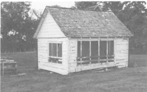
147) Chicken Coop Construction Date: ca. 1920 Location: SW 2-17-3E Present Owner: Mr. Hawkins Present Use: Storage Construction: walls - dovetailed logs roof - wood shingles on milled wooden rafters Integrity: Interior has been gutted Condition: Fair
