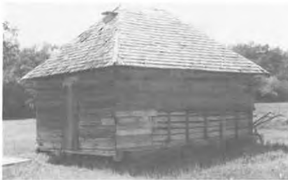
127) Log Granary Construction Date: ca. 1915 Location: River Lot #156 Present Owner: N. Schafer Present Use: Storage Construction: walls - horizontal siding on dovetailed logs roof - wood shingles on milled wooden rafters Integrity: Unaltered Condition: Good Notes: The hipped roof on this structure is unusual in the local context, where farmers preferred the simple gable roof.
