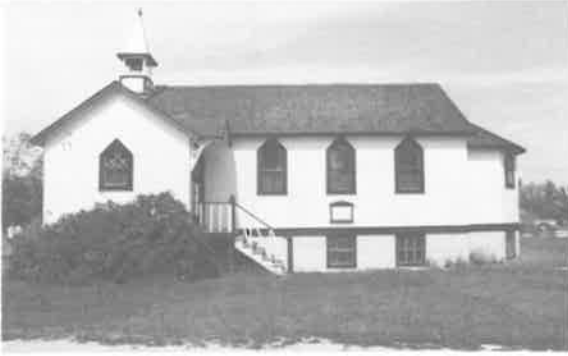
177) St. Peter's-Dynevor Church Construction Date: ca. 1925 Location: River Lot #34 Present Owner: Anglican Church of Canada Present Use: Active Congregation Construction: walls - horizontal siding on milled wooden frame roof - asphalt shingles on milled wooden rafters Integrity: Largely unaltered Condition: Good
