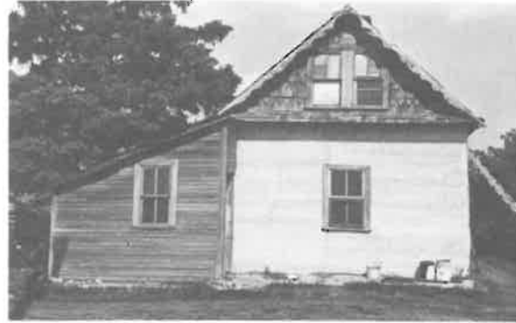
58) Galician Log House Construction Date: ca. 1920 Location: NW 12-17-3E Present Owner: Mr. Yakobowski Present Use: Occupied Construction: walls - plaster veneer on squared dovetailed logs roof - wood shingles on cut timbers Integrity: Largely unaltered Condition: Fair Notes: This building is also discussed on page 2 83-84.
