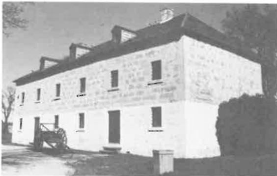
247) Warehouse Building Construction Date: 1830s Location: Lower Fort Garry National Historic Park Present Use: Display Construction: walls - dressed limestone roof - wood shingles on hewn timber rafters Integrity: The building has been carefully restored Condition: Good Notes: This building is also discussed on page 33.
