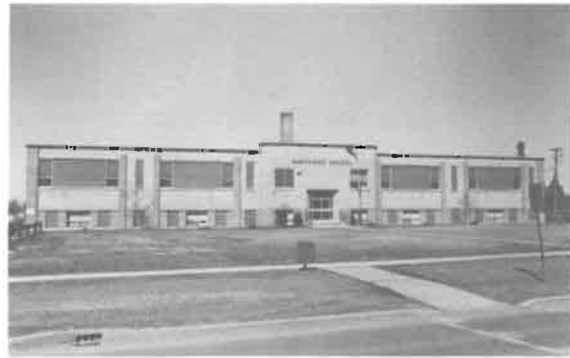
224) Daerwood School Construction Date: 1949 Location: Main Street, Selkirk Present Owner: Town of Selkirk Present Use: Active School Construction: walls - buff brick on milled wooden frame roof - built-up roofing Integrity: Largely unaltered Condition: Good
