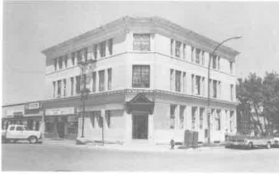
233) Former Dominion Bank Construction Date: ca. 1900 Location: Manitoba & Eveline, Selkirk Present Owner: Present Use: Various businesses and offices Construction: walls - buff brick on milled wooden frame roof - built-up tar and gravel Integrity: Both interior and exterior have been altered Condition: Good Notes: This building is also discussed on page 114.
