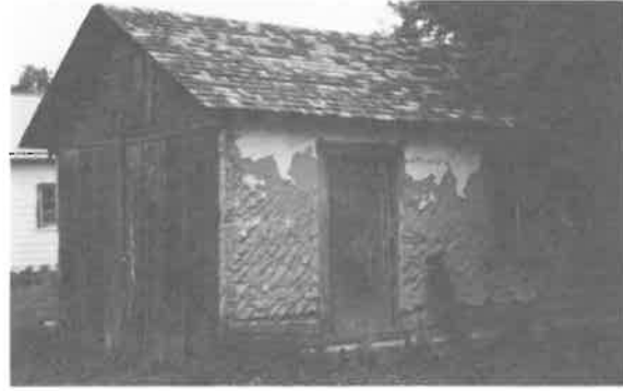
134) Machine Shed Construction Date: ca. 1930 Location: Present Owner: Peter Romanic Present Use: Storage Construction: walls - plaster and willow lath on dovetailed logs roof - wood shingles on milled wooden rafters Integrity: Largely unaltered Condition: Fair Notes: This building is also discussed on page 74.
