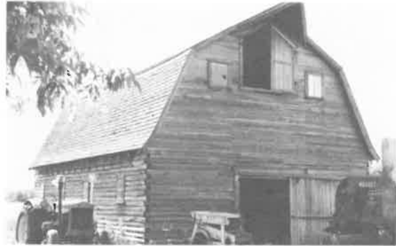
110) Log Barn Construction Date: ca. 1925 Location: SE 12-17-3E Present Owner: Mr. A. Husluk Present Use: Storage Construction: walls - pre-cut squared logs roof - wood shingles on milled wooden rafters Integrity: Unaltered Condition: Good
