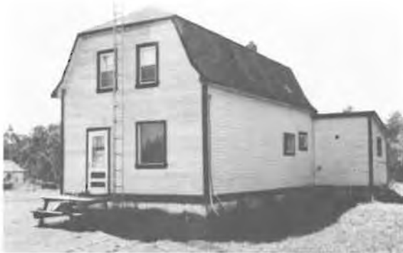
67) 1 1/2 Storey Side Hall House with Hipped Gable Roof Construction Date: ca. 1915 Location: NE 18-14-6E Present Owner: Manitoba Agricultural Credit Corporation Present Use: Occupied Construction: walls - horizontal siding on milled wooden frame roof - asphalt shingles on milled wooden rafters Integrity: Unaltered floorplan Condition: Good Notes: This building is also discussed on pages 58-59.
