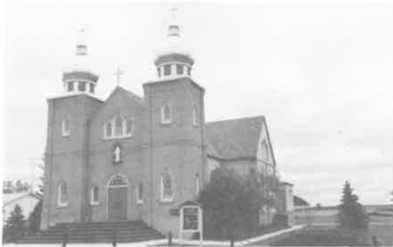
203) Holy Trinity Ukrainian Catholic Church Construction Date: 1952 Location: River Lots #201-204 Present Owner: Ukrainian Catholic Church of Canada Present Use: Active Congregation Construction: walls - stucco veneer on milled wooden frame roof - asphalt shingles on milled wooden rafters Integrity: Largely unaltered Condition: Good Notes: This building is also discussed on page 100.
