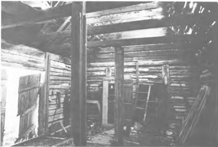
Plate 22. The interior of the barn at SW10-14-4E reveals the beaded beams and the differently finished wall logs -- the lower ones are squared, the upper ones are left rounded -- that suggest the structure was composed of pieces from several buildings.
