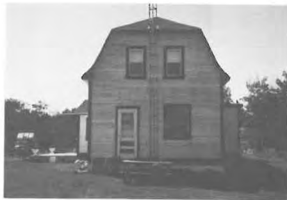
Plate 78. The hipped gambrel roof on this house is distinctive.
