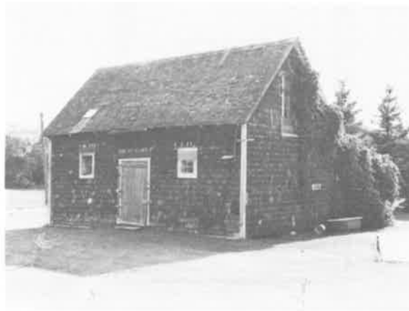
Plate 70. Hawkins house at SW12-17-3E, a typical log structure of the 1880s within the planning area.
