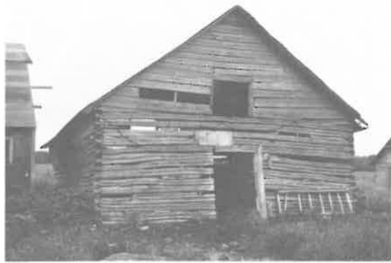
Plate 138. Former Gabryk barn.
