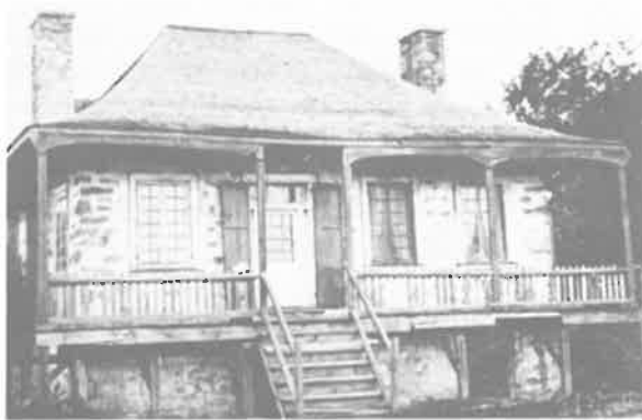
Plate 34. The distinctive bellcast roof and verandah of Quebec houses are evident here. (From: The Old Architecture of Quebec , p. 64.)
