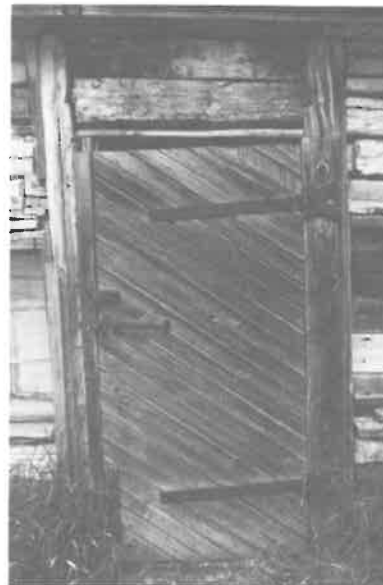
Plate 19. The original hand-forged locks and hinges were used on the reconstruction of the Kuhn barn.
