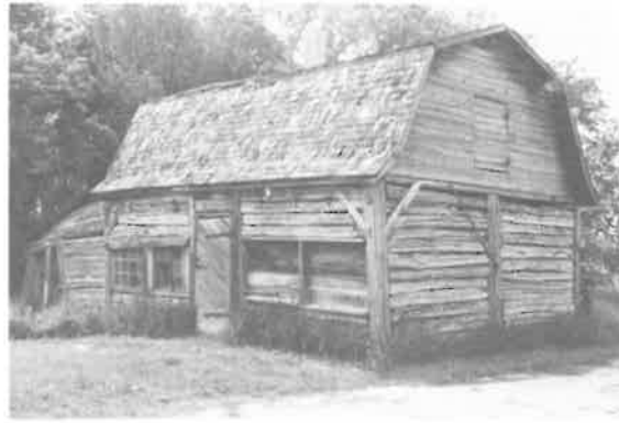
Plate 18. Kuhn barn, just south of Lower Fort Garry.
