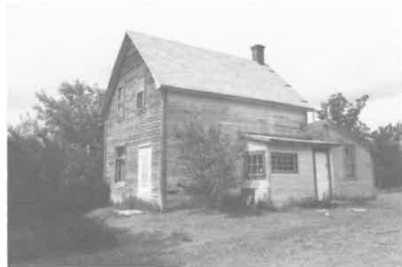
Plate 73. Former MacArthur house, near Little Britain.
