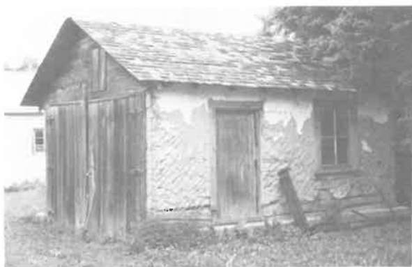
Plate 106. Log machinery shed, SE34-13-3E.
