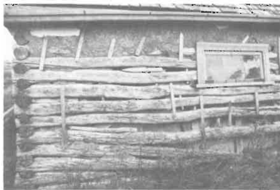
Plate 141. This detail of a granary shows the long pegs used to secure the walls against lateral spread.
