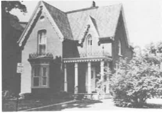
Plate 63. An L-shaped plan gives this 1875 Gothic Revival house in Hamilton variety and a sense of the picturesque. (From: Gothic Revival in Canadian Architecture , p. 149.)
