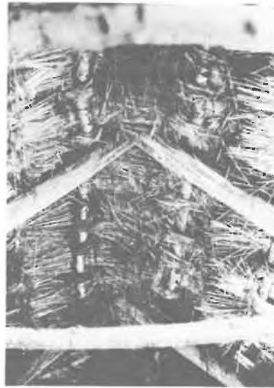
Plate 126. Thatch procedure likely used on the former Arnsey house.
