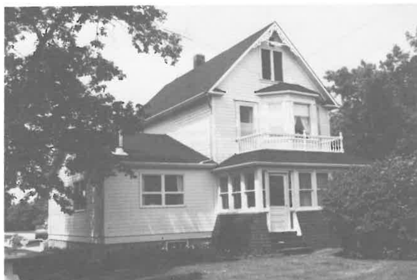
Plate 76. This side hall house, just north of Little Britain United Church, was treated with several details, including bay windows, a verandah, window surrounds and a small delicate bargeboard.
