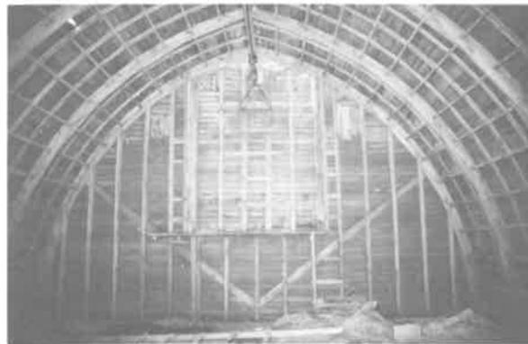
Plate 98. Detail of typical rafter construction in a vaulted loft.
