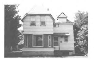
l l/2 Store L-Shaped House Construction Date: ca. 1895 Location: 204 Taylor Avenue, Selkirk Present Owner: G. E. Still Present Use: Occupied Construction: walls - aluminum siding on milled wooden frame roof - asphalt shingles on milled wooden rafters Inregrity: Both interior and exterior have been significantly altered. Condition: Good
