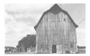
Large Light Wood Frame Barn Construction Date: 1912 Location: River Lot #20 Present Owner: Mr. Overwater Present Use: Storage Construction: walls - concrete stable and light frame loft roof - wood shingles on built-up wooden rafters Integrity: Unaltered Condition: Good Notes: This building is also discussed on pages 65-66.
