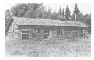
Chicken Coop Construction Date: ca. 1920 Location: SE 22-16-3E Present Owner: A. Dalman Present Use: Abandoned Construction: walls - horizontal siding on milled wooden frame roof - wood shingles on milled wooden rafters Integrity: Unaltered Condition: Poor Notes: This building is also discussed on page 75.
