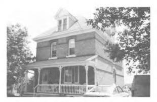
2 1/2 Storey Square Plan House Construction Date: 1911 Location: 478 Eveline Street, Selkirk Present Owner: Mr. G. McLeod Present Use: Occupied Construction: walls - red brick on milled wooden frame roof - asphalt shingles on milled wooden rafters Integrity: Largely unaltered Condition: Good Notes: This building is also discussed on page 120.
