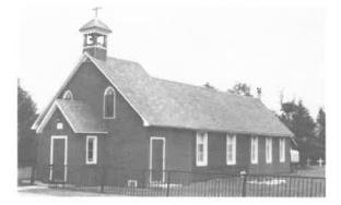
194) St. Anne's Polish Catholic Church Construction Date: 1934 Location: Petersfield Present Owner: Polish Catholic Church of Canada Present Use: Active Congregation Construction: walls - insulbrick siding on milled wooden frame roof - asphalt shingles on milled wooden rafters Integrity: Largely unaltered
