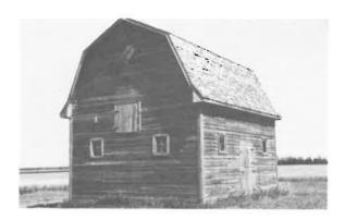
111) Small Light Wood Frame Barn Construction Date: ca. 1925 Location: SW 21-15-6E Present Owner: Present Use: Storage Construction: walls - horizontal siding on milled wooden frame
