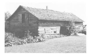
120) Log Barn Construction Date: 1943 Location: NW 10-17-7E Present Owner: Mr. K. Klatt Present Use: Vacant Construction: walls - squared dovetailed logs roof - wood shingles on milled wooden rafters Integrity: Unaltered Condition: Fair
