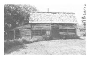
94) Log Barn Construction Date: 1860 (reconstructed 1922) Location: River Lot #129 Present Owner: Mr. P. Kuhn Present Use: Storage Construction: walls - Red River Frame log construction roof - wood shingles on milled wooden rafters Integrity: The barn was once much larger and oriented differently. Materials from the 1860 barn were used in this barn. Condition: Poor
