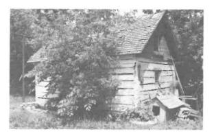
154) Summer Kitchen Construction Date: 1926 Location: River Lot #240 Present Owner: E. Huzarski Present Use: Storage Construction: walls - dovetailed logs roof - wood shingles on milled wooden rafters Integrity: Interior has been gutted Condition: Fair
