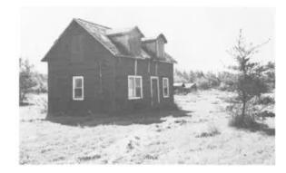
84) 1 I/2 Storey Central Plan House Construction Date: ca. 1930 Location: NE 32-16-7E Present Owner: Mr. A. Hourie Present Use: Vacant Construction: wells - insulbrick veneer on milled wooden frame roof - wood shingles on milled wooden rafters Integrity: Largely unaltered Condition: Poor
