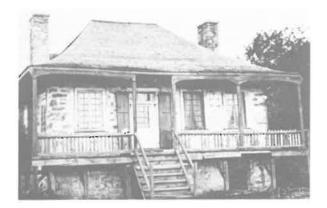
Plate 34. The distinctive bellcast roof and verandah of Quebec houses are evident here. (From: The Old Architecture of Quebec, p. 64.)
