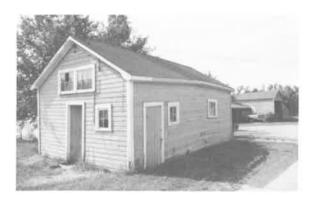
142) Shed Construction Date: 1915 Location: SE 1-15-4E Present Owner: Mr. Macklin Present Use: Storage Construction: walls - horizontal siding on milled wooden frame roof - asphalt shingles on milled wooden rafters Integrity: Unaltered Condition: Good
