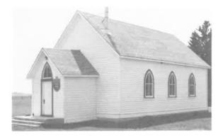
Dunara United Church Construction Date: 1893 Location: SE 36-15-3E Present Owner: United Church of Canada Present Use: Active Congregation Construction: walls - herizontal siding on milled wooden frame roof - asphalt shingles on milled wooden rafters Integrity: Largely unaltered Condition: Good
