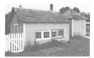
149) Chicken Coop Construction Date: ca. 1915 Location: River Lot #82 Present Owner: Mr. Goltz Present Use: Storage Construction: walls - horizontal siding on milled wooden frame roof - wood shingles on milled wooden rafters Integrity: Unaltered Condition: Good
