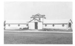
146) Bunkhouse/Machine Shed Construction Date: ca. 1925 Location: NE 2-16-3E Present Owner: C.P. Kollar Present Use: Storage Construction: walls - horizontal siding on milled wooden frame roof - wood shingles on milled wooden rafters Integrity: The attached wings have been altered to accommodate larger machinery Condition: Good
