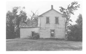
1 1/2 Storey L-Shaped House Construction Date: ca. 1900 Location: SE 3-15-4E Present Owner: H. Zelyk Present Use: Vacant Construction: walls - horizontal siding on milled wooden frame roof - wood shingles on milled wooden rafters Integrity: Largely unaltered Condition: Poor
