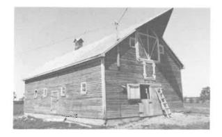
109) Large Light Wood Frame Barn Construction Date: ca. 1920 Location: NE. 18-16-8E Present Owner: G. Lloyd Present Use: Functioning Barn Construction: walls - horizontal siding on milled wooden frame roof - metal sheeting on milled wooden rafters Integrity: Unaltered Condition: Good
