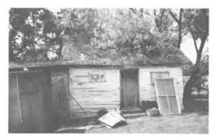
97) Heavy Wood Frame Barn Construction Date: ca. 1910 Location: NW 24-15-6E Present Owner: Mr. C. Horbady Present Use: Storage Construction: walls - horizontal and vertical siding on heavy wood frame roof - wood shingles on milled wooden rafters
