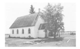
172) St. Matthew's Anglican Church Construction Date: 1906 Location: SW 33-I3-4E Present Owner: Anglican Church of Canada Present Use: Active Congregation Construction: walls - horizontal siding on milled wooden frame roof - wood shingles on milled wooden rafters Integrity: Largely unaltered Condition: Good Notes: This building is also discussed on pages 94-95.
