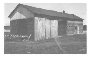
Light Wood Frame Barn Construction Date: ca. 1930 Location: NE 30-16-8E Present Owner: Mr. F. Klann Present Use: Storage/Granary Construction: walls - horizontal aiding on milled wooden frame roof - asphalt shingles on milled wooden rafters Integrity: Unaltered Condition: Fair Notes: This building is also discussed on page 74.
