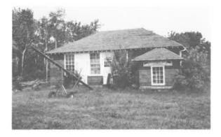
221) Brookside School Construction Date: ca. 1925 Location: SE II-14-5E Present Owner: W. Jacyk Present Use: Storage Construction: walls - insulbrick veneer on milled wooden frame roof - asphalt shingles on milled wooden rafters Integrity: Unaltered Condition: Good
