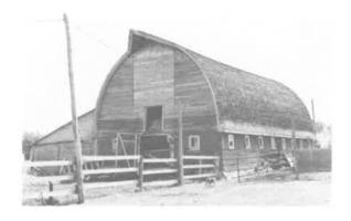
Large Light Wood Frame Barn with Vaulted Roof Construction Date: ca. 1940 118) Location: SW 9-14-4E Present Owner: Mr. T. Jenkins Present Use: Functioning Barn Construction: walls - horizontal siding on milled wooden frame roof - wood shingles on built up rafters Integrity: The stable has been altered to produce a more open space Condition: Fair Notes: This building is also discussed on pages 69-70.
