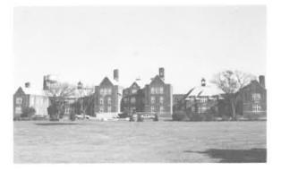
238) Reception Hospital Construction Date: 1922 Location: Selkirk Mental Health Centre Present Owner: Selkirk Mental Health Centre Present Use: Functioning Hospital Construction: walls - red brick veneer on milled wooden frame roof - asphalt shingles on sloped surfaces; built-up roofing on flat surfaces Integrity: Largely unaltered Condition: Good Notes: This building is also discussed on page 113.
