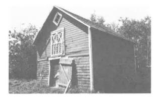
117) Small Light Wood Frame Barn Construction Date: 1938 Location: SE 7-14-6E Present Owner: Mr. M. Chorney Present Use: Storage Construction wells - horizontal siding on milled wooden frame roof - wood shingles on milled wooden rafters Integrity: Stable has been altered
