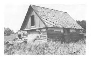
Log Granary Construction Date: ca. 1910 126) Location: Present Owner: Present Use: Vacant Construction: walls - dovetailed logs with plaster cover roof - wood shingles on milled wooden rafters Integrity: Unaltered, but plaster is disintegrating Condition: Fair
