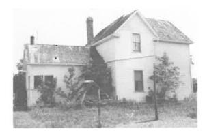
1 1/2 Storey L-Shaped House Construction Date: 1900 Location: SW 9-14-4E Present Owner: T. Jenkins Present Use: Storage Construction: walls - horizontal siding on milled wooden frame roof - wood shingles on milled wooden rafters Integrity: Largely unaltered Condition: Good
