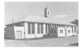
241) Leundry Building Construction Date: 1920 Location: Selkirk Mental Health Centre Present Owner: Selkirk Mental Health Centre Present Use: Laundry facility Construction: walls - stucco veneer on milled wooden frame roof - asphalt shingles Integrity: Largely unaltered Condition: Good
