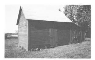
Granary Construction Date: ca. 1930 Location: SW 27-15-6E Present Owner: Present Use: Storage Construction: walls - horizontal siding on milled wooden frame roof - wood shingles on milled wooden rafters Integrity: Unaltered Condition: Good
