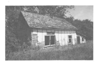
Log House Construction Date: ca. 1920 Location: River Lot #151 Present Owner: Present Use: Vacant Construction: walls - plaster veneer on squared dovetailed logs roof - wood shingles on cut timbers Integrity: Largely unaltered Condition: Poor Notes: This building is also discussed on page 85.
