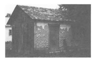
Machine Shed Construction Date: ca. 1930 Location: Present Owner: Peter Romanic Present Use: Storage Construction: walls - plaster and willow lath on dovetailed logs roof - wood shingles on milled wooden rafters Integrity: Largely unaltered Condition: Fair Notes: This building is also discussed on page 74.
