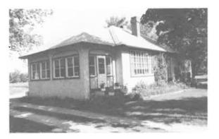
86) Single Storey House Construction Date: ca. 1920 Location: River Lot #10 Present Owner: Mr. John Grochowich Present Use: Occupied Construction walls - stucco veneer on milled wooden frame roof - asphalt shingles on milled wooden rafters Integrity: Largely unaltered Condition: Good Notes: This building was constructed as a summer cottage by a former manager of Eaton's Department Store in Winnipeg. A garage and chauffeur's quarters are at the back of the site.
