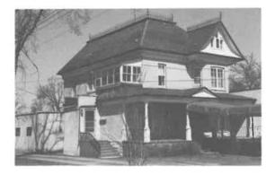
29) 2 1/2 Storey Square Plan House Construction Date: 1913 Location: 307 Eveline Street, Selkirk Present Owner: Mr. Roy Gilbart Present Use: Funeral Parlour Construction: walls - buff brick on milled wood frame roof - wood shingles on milled wooden rafters Integrity: The interior has been altered considerably.
