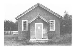
222) Stony Point School Construction Date: ca. 1925 Location: SE 6-17-7E Present Owner: R.M. of St. Clements Present Use: Vacant Construction: walls - insublrick veneer on milled wooden frame roof - asphalt shingles on milled wooden rafters Integrity: Unaltered Condition: Poor
