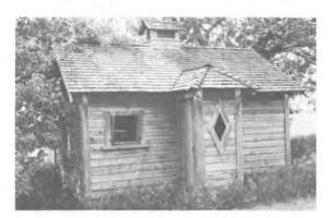
162) Outhouse Construction Date: ca. 1920 Location: Present Owner: Present Use: Vacant Construction: walls - horizontal siding on milled wooden frame roof - wood shingles on milled wooden rafters Integrity: Unaltered Condition: Good
