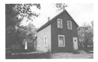
62) 1 1/2 Storey Side Hall House Construction Date: ca. 1905 Location: River Lot #97 Present Owner: M. Clark Present Use: Occupied Construction: wells - insulbrick siding on milled wooden frame roof - wood shingles on milled wooden rafters Integrity: Largely unaltered Condition: Fair
