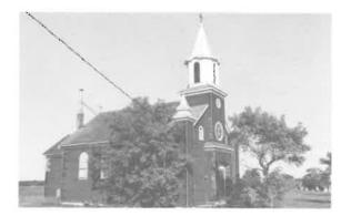
198) Sacred Heart Chapel, Victoria Park Construction Date: 1937 Location: River Lot #70 Present Owner: Present Use: Vacant Construction: walls - insulbrick siding on milled wooden frame roof - wood shingles on milled wooden rafters Integrity: Largely unaltered Condition: Poor Notes: This building has been dismantled and the hall section used as a private residence.
