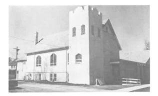
182) Selkirk United Church Construction Date: 1986 Location: 202 McLean Avenue, Selkirk Present Owner: United Church of Canada Present Use: Active Congregation Construction: Walls - stucco on milled wooden frame roof - asphalt shingles on milled wooden rafters Integrity: The building originally stood on Dufferin Avenue. Condition: Good
