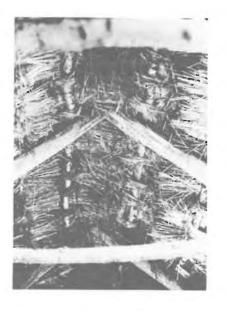
Plate 126. Thatch procedure likely used on the former Arnsey house.
