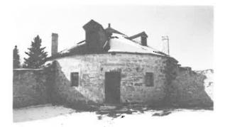
250) Southwest Bastion Construction Date: 1840s Location: Lower Fort Garry National Historic Park Present Owner: Parks Canada Present Use: Display Construction: walls - dressed limestone roof - wood shingles on hewn timber rafters Integrity: The structure has been carefully restored.
