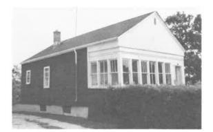
30) Single Storey House Construction Date: ca. 1880 Location: 515 Clandeboye Avenue, Selkirk Present Owner: Mr. K. Davidson Present Use: Occupied Construction: walls - insulbrick siding on milled wooden frame roof - asphalt shingles on milled wooden rafters Integrity: Unaltered floorplan
