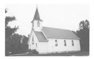
190) St. John's Evengelical Lutheran Church Construction Date: ca. 1920 Location: SW 19-15-8E Present Owner: Lutheran Church of Canada Present Use: Active Congregation Construction: walls - horizontal siding on milled wooden frame roof - asphalt shingles on milled wooden rafters Integrity: Largely unaltered Condition: Good
