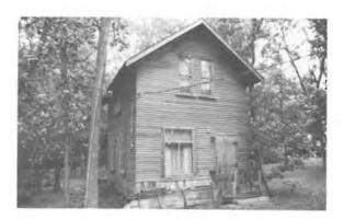
1 1/2 Storey Side Hall House Construction Date: ca. 1915 Location: River Lot #117 Present Owner: Mr. C. Douglas Present Use: Vacant Construction: walls - horizontal siding on milled wooden frame roof - asphalt shingles on milled wooden rafters Integrity: Largely unaltered Condition: Good
