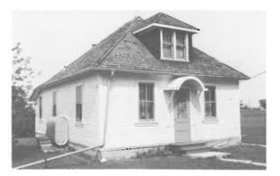
1 I/2 Storey Cottage Construction Date: 1929 Location: River Lot #242 Present Owner: Mrs. Zybyluk Present Use: Occupied Construction: walls - horizontal siding on milled wooden frame roof - wood shingles on milled wooden rafters Integrity: Largely unaltered Condition: Good
