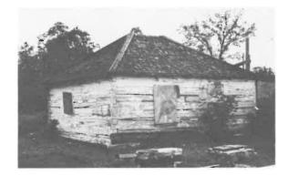
Log House Construction Date: 1931 Location: SE 6-17-7E Present Owner: Mr. W. Viznagh Present Use: Storage Construction: walls - squared dovetailed logs roof - wood shingles on milled wooden rafters Integrity: Largely unaltered Condition: Fair
