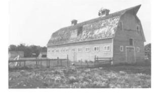
Large Light Wood Frame Barn Construction Date: 1915 Location: SE 1-15-4E Present Owner: Mr. Macklin Present Use: Functioning Barn Construction: walls - horizontal siding on milled wooden frame roof - wood shingles on milled wooden rafters Integrity: Unaltered
