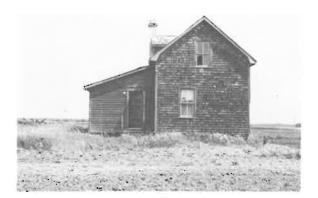
81) 1 I/2 Storey House Construction Date: ca. 1925 Location: SW 23-16-3E Present Owner: R. Penner Present Use: Vacant Construction: walls - wood shingles on milled wooden frame roof - wood shingles on milled wooden rafters Integrity: Largely unaltered Condition: Fair
