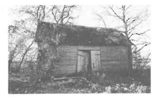
P3) Red River Frame Barn Construction Date: ca. 1870 Location: SW 10-14-4E Present Owner: Present Use: Vacant Construction: walls - Red River frame logs roof - wood shingles on hewn log rafters Integrity: Largely unaltered Condition: Poor Notes: This building is one of only three remaining structures in the planning area that used Red River frame construction procedures.
