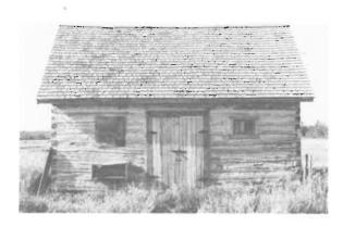
123) Log Granary Construction Date: ca. 1930 Location: Present Owner: Arnold Husluk Present Use: Storage Construction: walls - dovetailed squared logs roof - wood shingles on hewn log rafters Integrity: Unaltered Condition: Good Notes: This building is also discussed on page 71.
