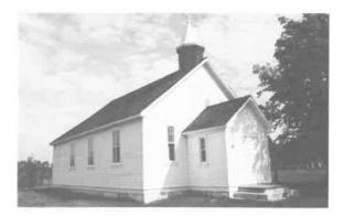
210) Libau Lutheran Church Construction Date: ca. 1920 Location: Libau Present Owner: Lutheran Church of Canada Present Use: Active Congregation Construction: walls - horizontal siding on milled wooden frame roof - wood shingles on milled wooden rafters Integrity: Largely uneltered Condition: Good Notes: This building is also discussed on page 128.
