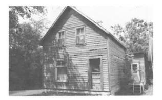
61) 1 1/2 Storey Side Hall House Construction Date: ca. 1905 Location: River Lot #255 Present Owner: S. Michaelson Present Use: Vacant Construction: walls - horizontal siding on milled wooden frame roof - asphalt shingles on milled wooden rafters Integrity: Largely unaltered Condition: Fair
