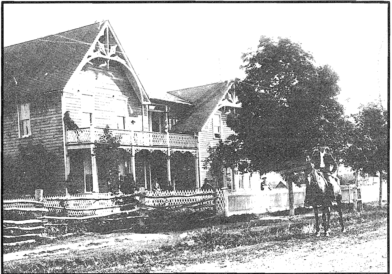
Residence of James Colcleugh, c.1888
