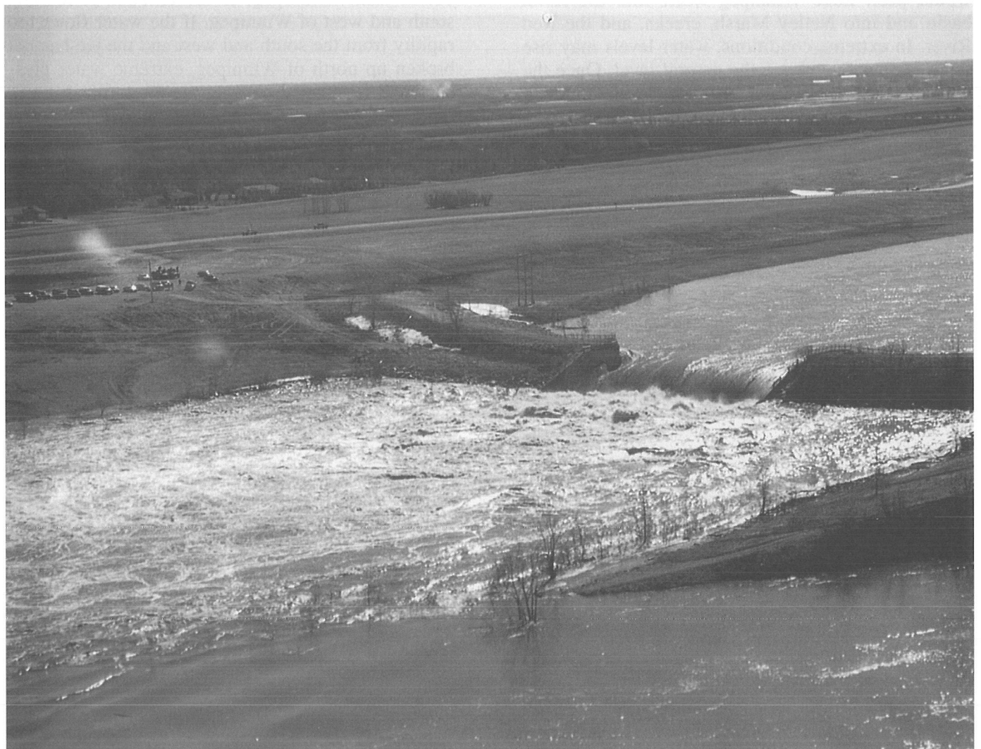
Floodway at Lockport, 1997.
