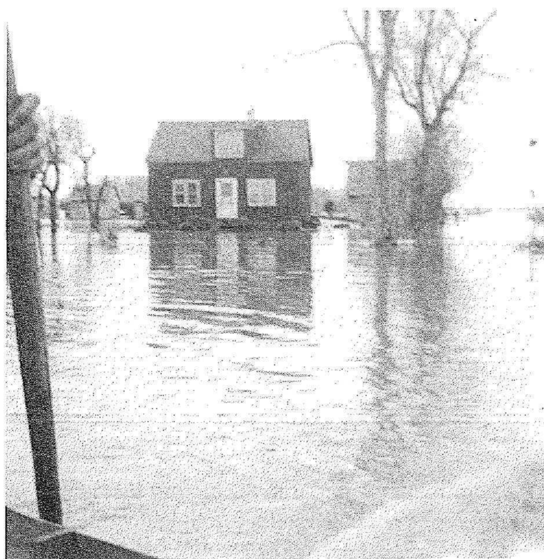
Walter Zador's residence (old Chyborak place) Breezy Point, Spring flood April 9-11, 1966.
