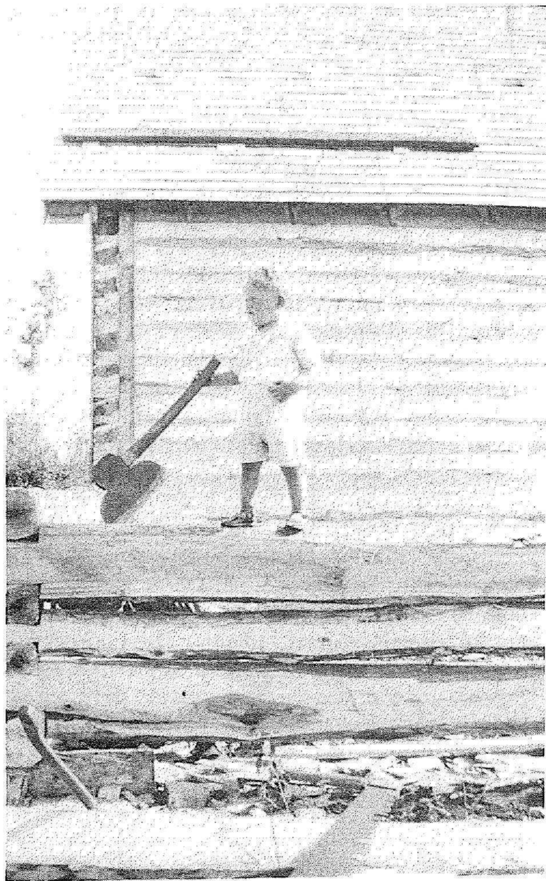
Roy Taylor's log house under construction with son Ross, "manning" the broadaxe, 1933.
