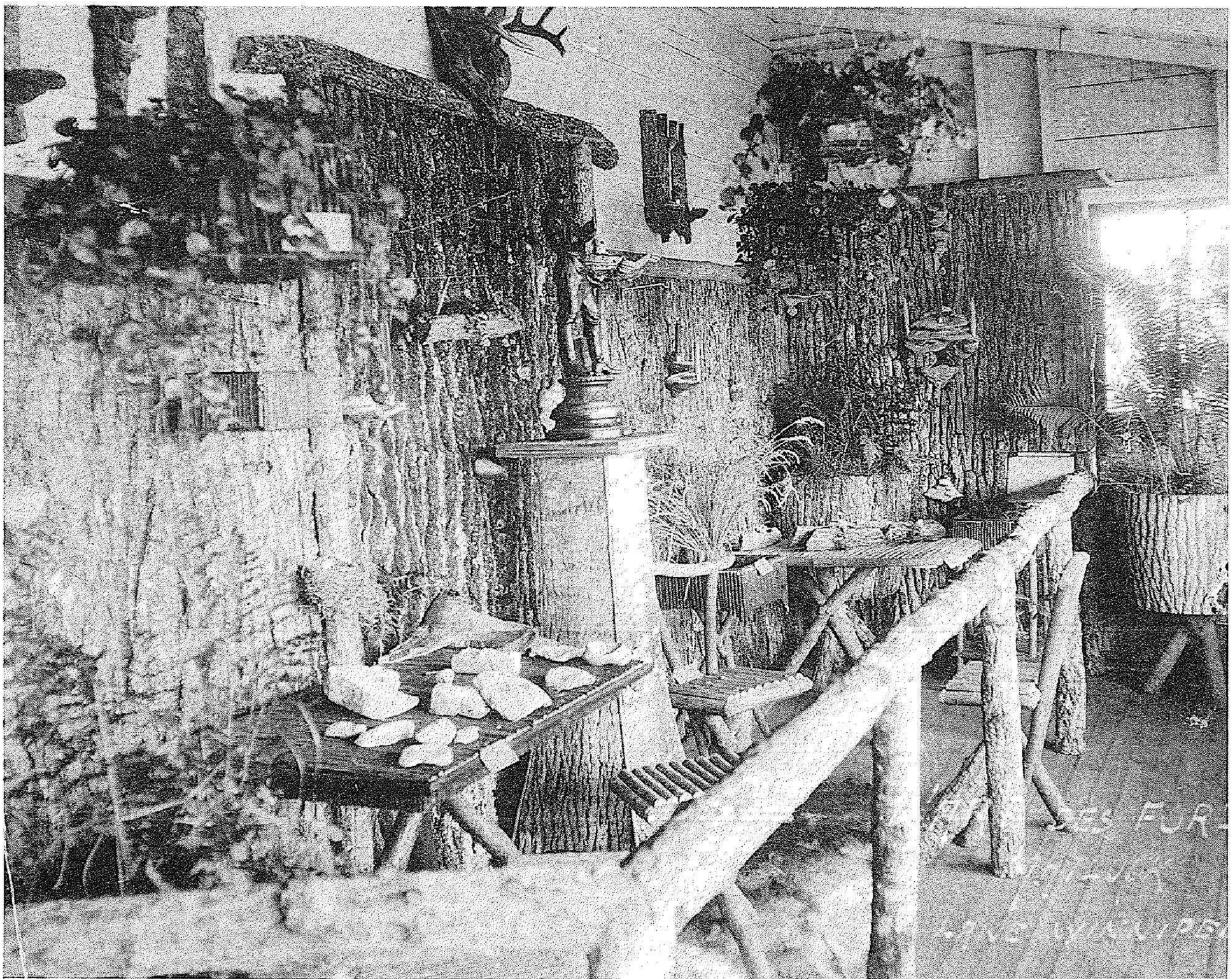
Tea Room, Matlock store. All wood furniture construction by J. O. Collede and helpers.
