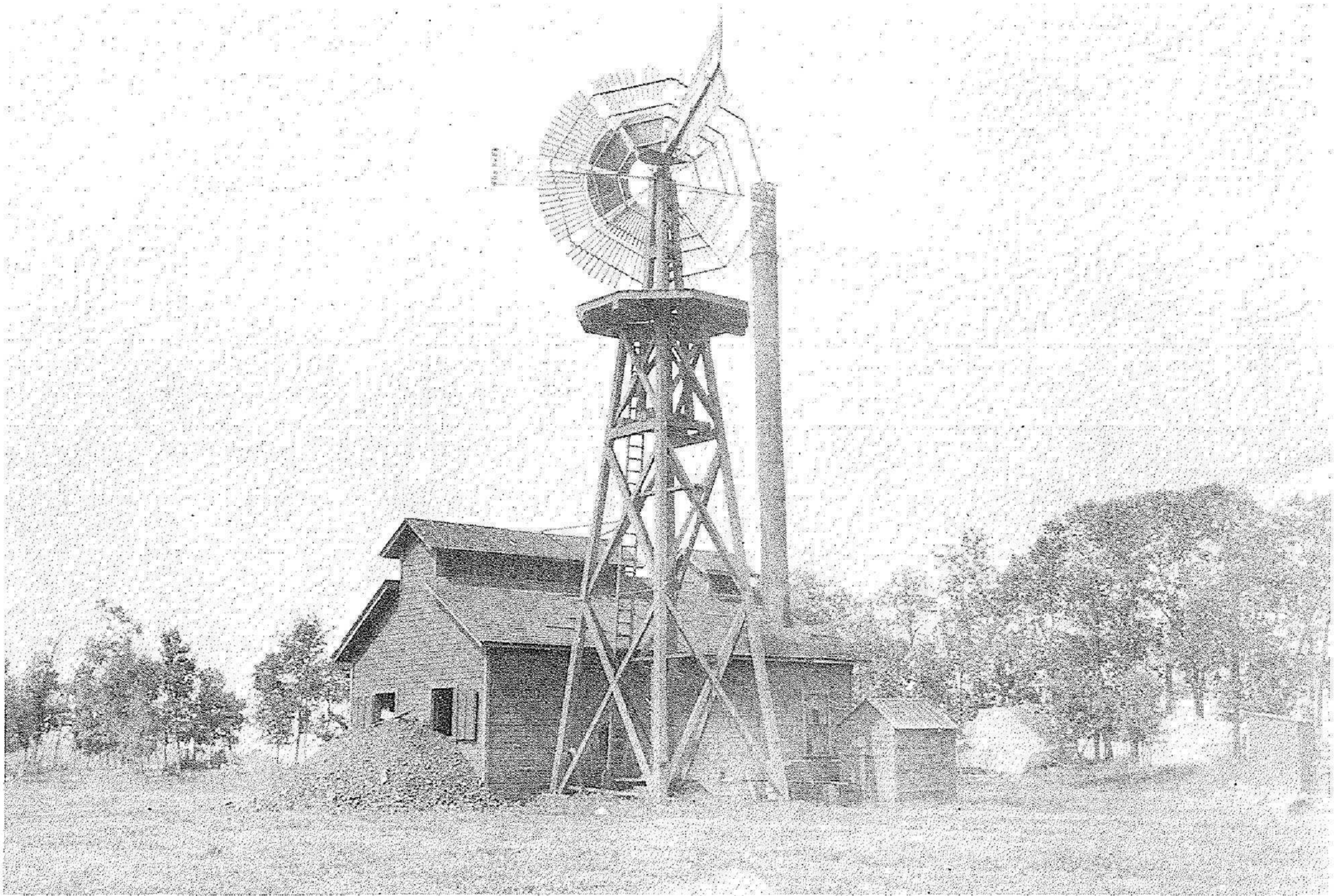
Power House, Winnipeg Beach, Circa 1915.
