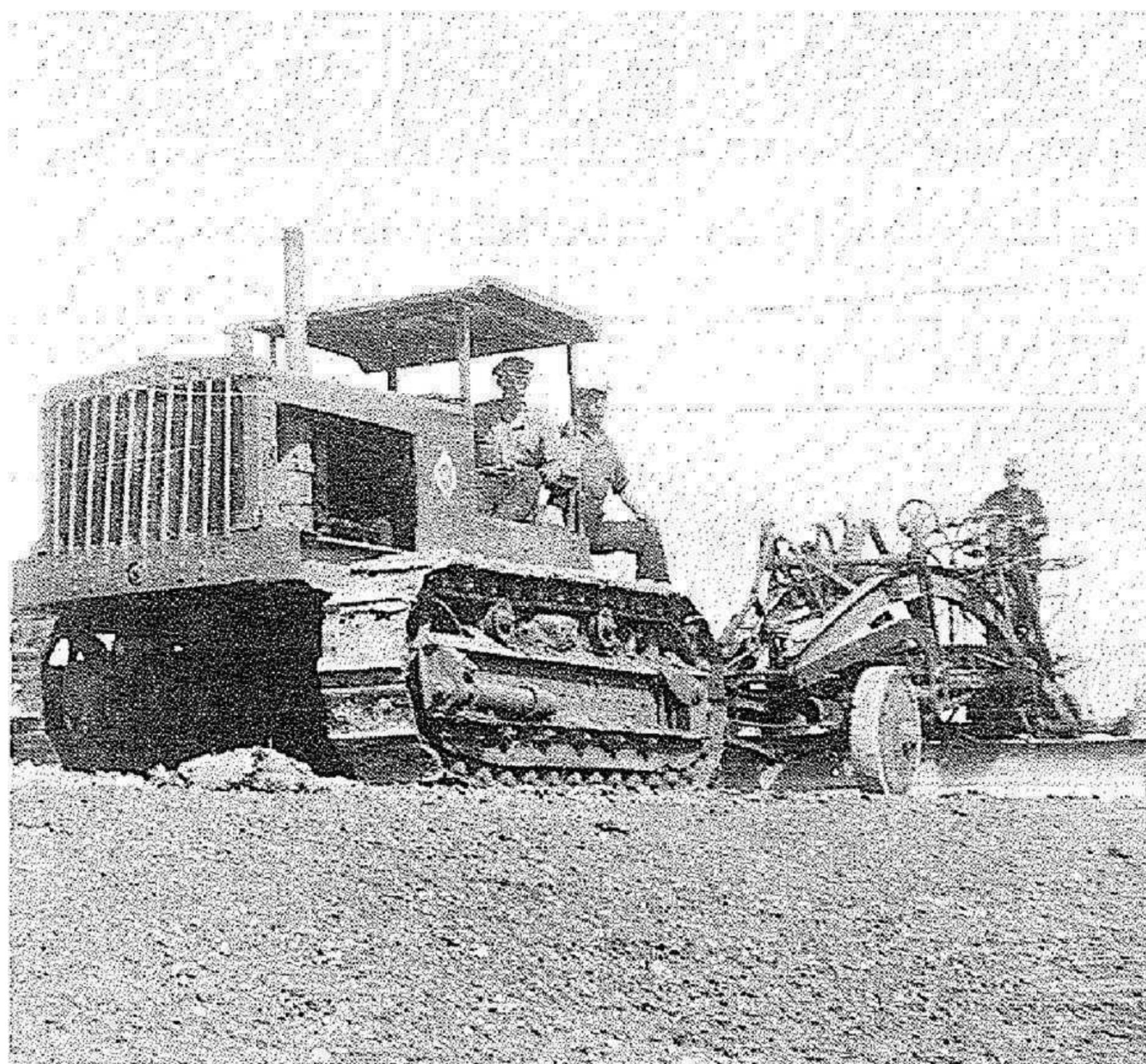
Municipal road maintenance, 1933. Alex Gunn on tractor and Bill Junior on grader.
