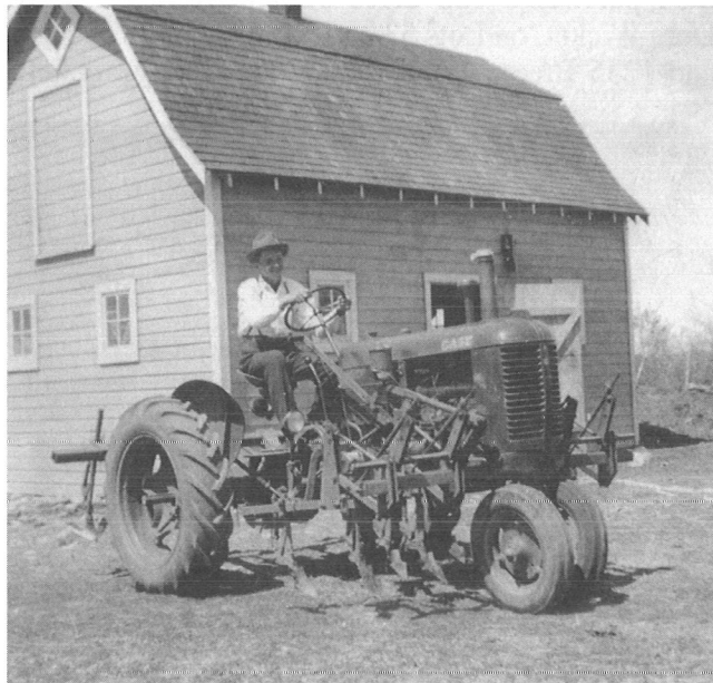
Row crop tractor with cultivator attachment.
