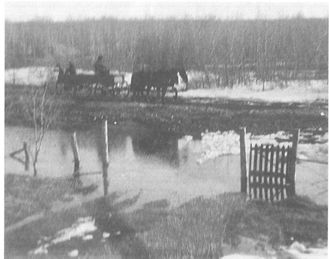
Flooded ditch on St. Andrew's Road in 1923 – now PTH 410.
