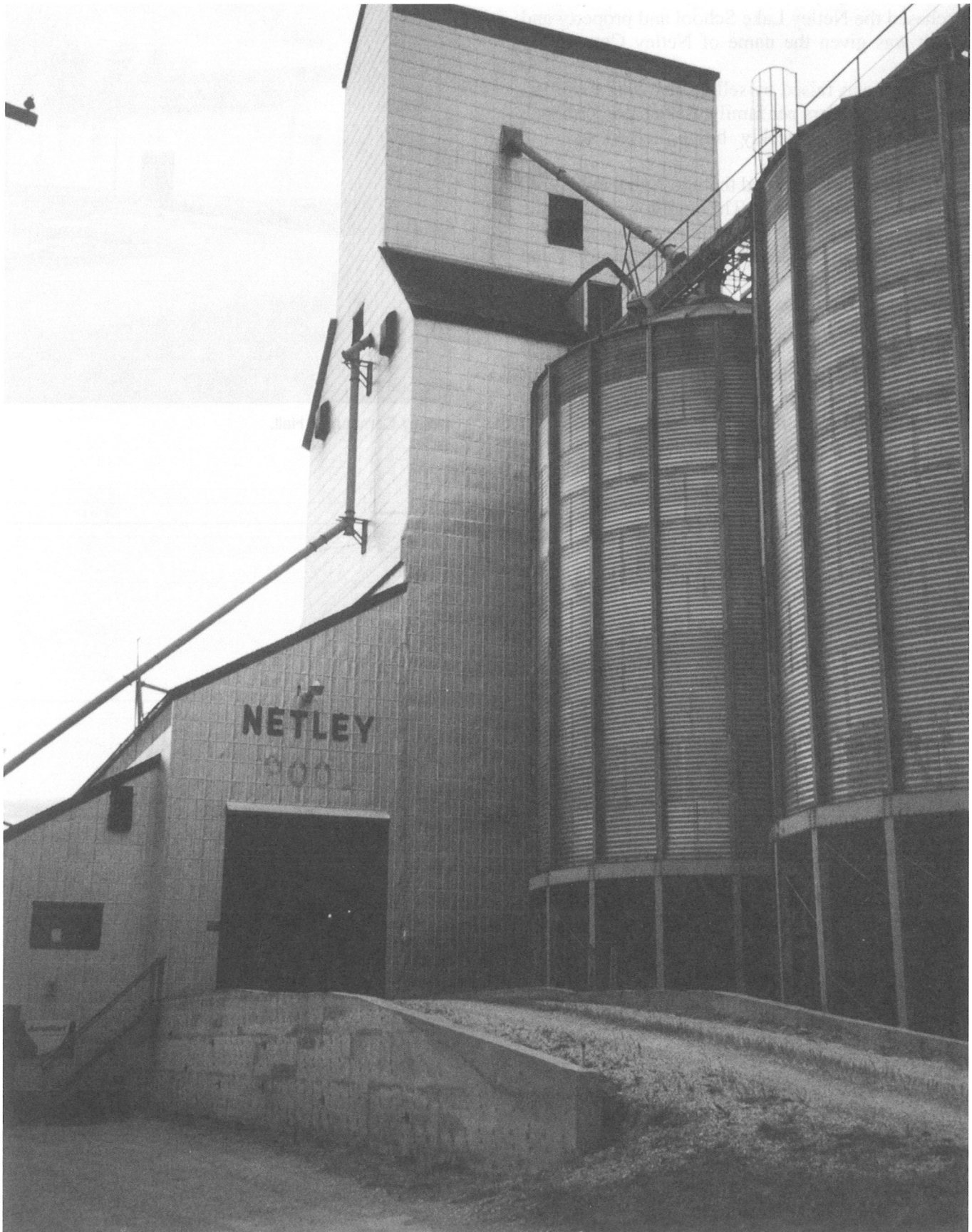
Entrance to grain elevator and terminal at Netley.
