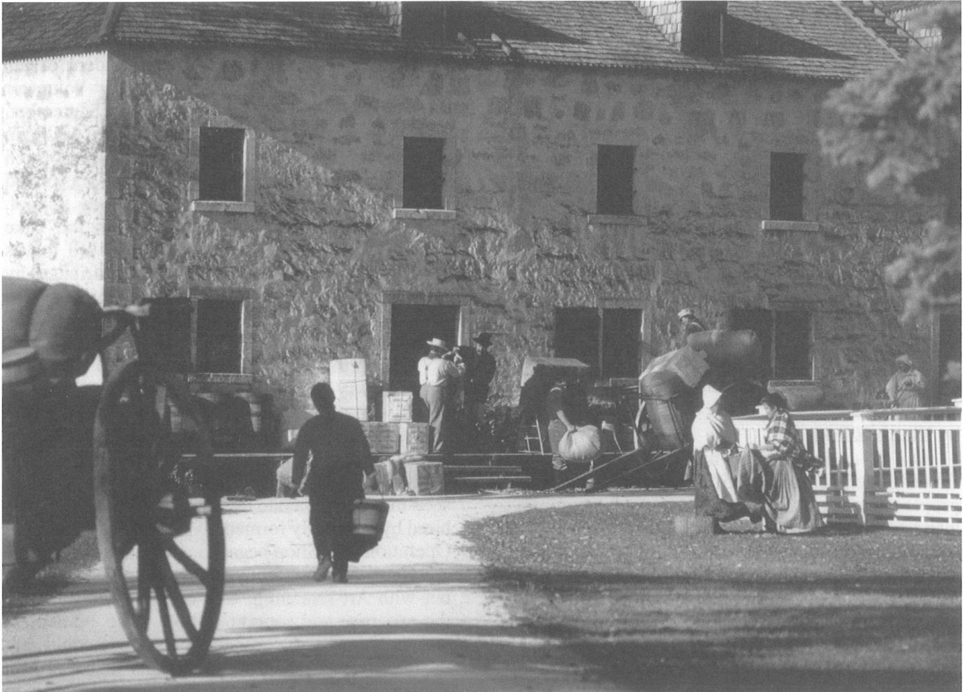
Lower Fort Garry fur loft and sales shop.
