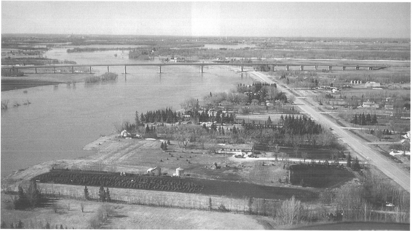
St. Peters Dynevor Bridge on #4 Hwy, 1997.
