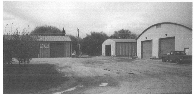
St. Andrews Central Fire Hall and municipal sheds.
