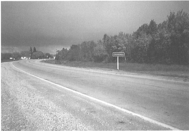
Approaching Clandeboye from the south on Hwy #9.
