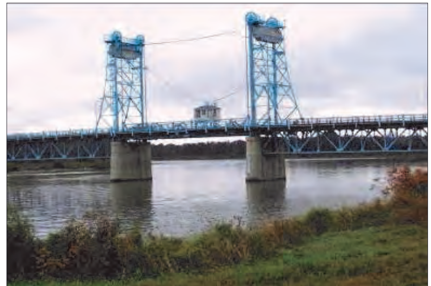
Selkirk Lift Bridge
