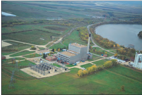
Selkirk Generating Station
