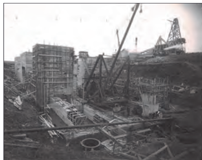
Lock and Dam construction
