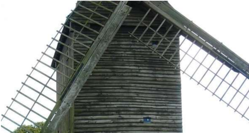
View of the kind of lattice-work that defined many windmill sail compositions.
