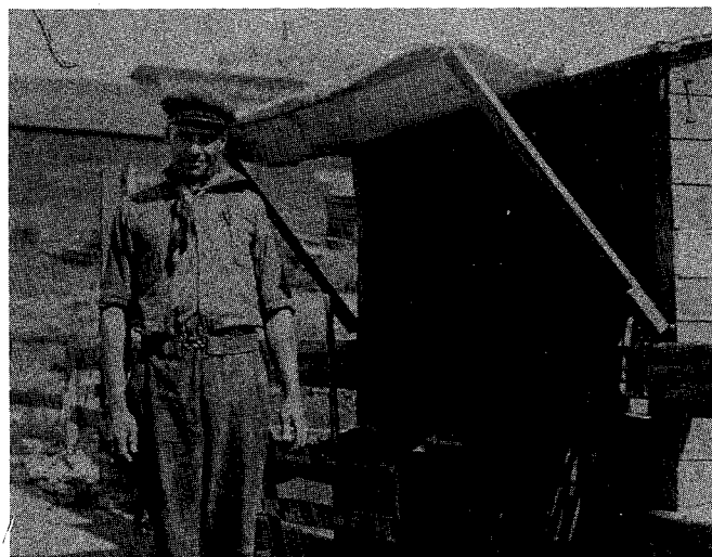
Fred Kordalchuk at the East Selkirk Ferry Dock.
