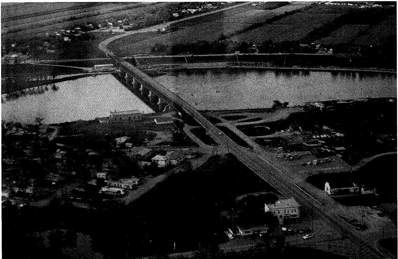
Lockport Corner, East Approach
