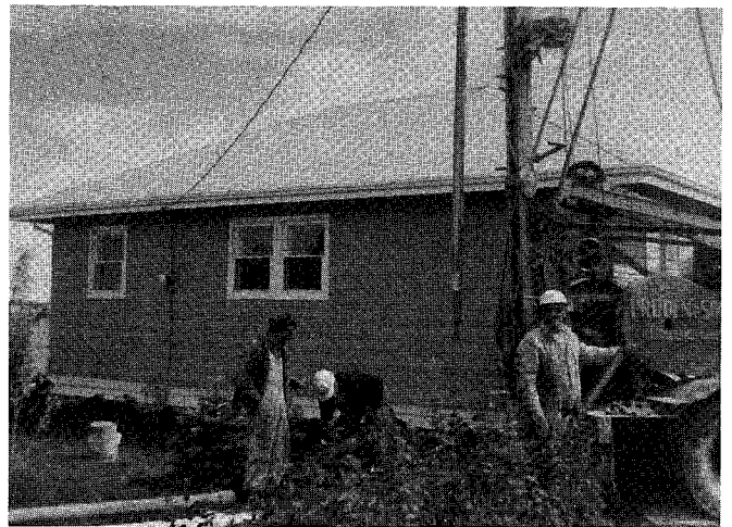
Charlie Pruden drilling in Libau west of the Libau hotel.
