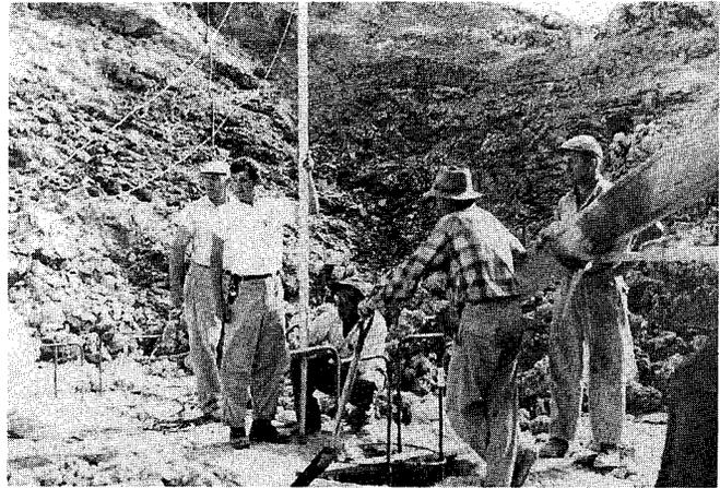
*Selkirk Generating Station Project: Levels are checked prior to pouring the concrete, 1957.*
