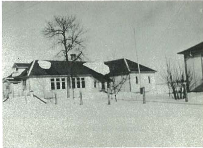
Donald School North building and South building two classrooms each.
