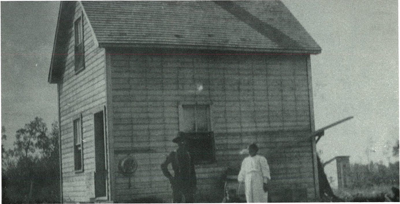
Hick's residence near the Quarry in East Selkirk served as the East Selkirk School and Meeting place.
