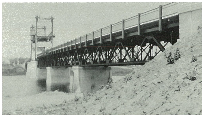
Selkirk Bridge on July 9, 1936.
