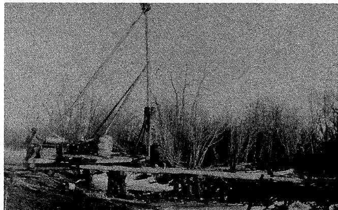
Long Bridge - driving piles.
