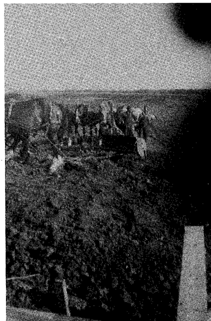
St. Peters Road building in 1946.
