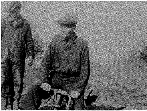
Road construction in 1937 - Art Boulton on Jackhammer.
